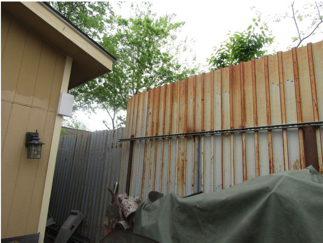
12' Rear Yard Fence with Corrugated Metal Fence Material
