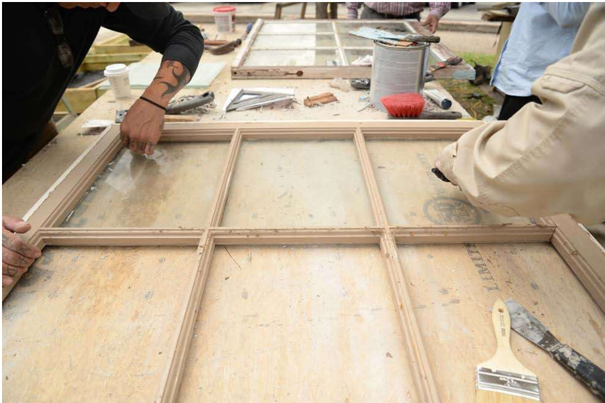
Historic wood frames are restored, and prepped for reglazing.
