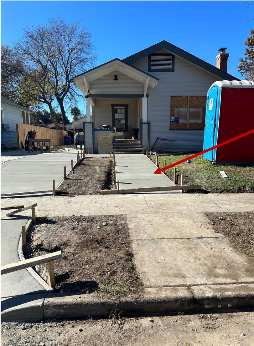
This sidewalk was there already but broken up. It was cleaned up and flattened for wheelchair access.
