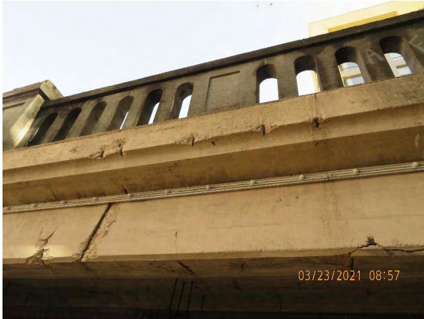
*Figure 12: Typical minor spalling along southern overhang*
