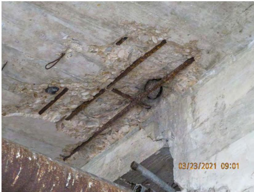
*Figure 13: Major spalling with exposed reinforcing in deck between southernmost beams 1 & 2*
