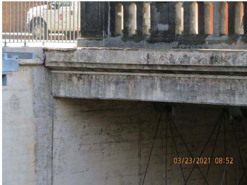
*Figure 5: Typical moderate spalling with exposed reinforcing at exterior north beam*
