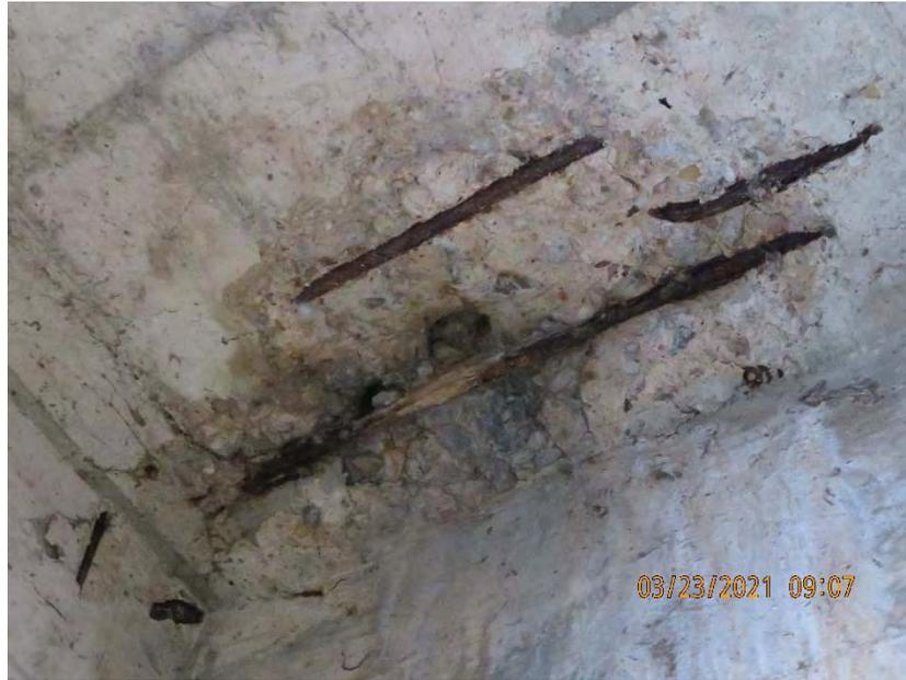
*Figure 14: Major spalling with exposed reinforcing in deck between northernmost beams 2 & 3*
