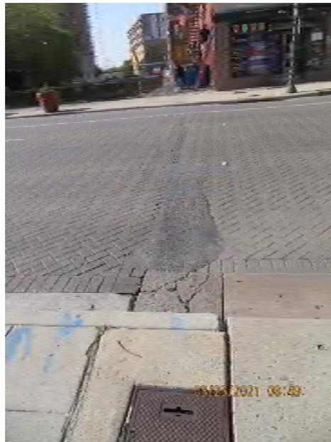
*Figure 19: Differential settlement and rutting at abutment joints*
