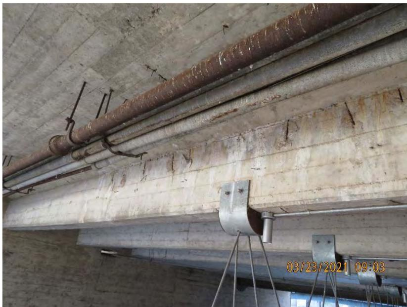
*Figure 22: Multiple utilities and pedestrian bridge suspended from slab & beams*
