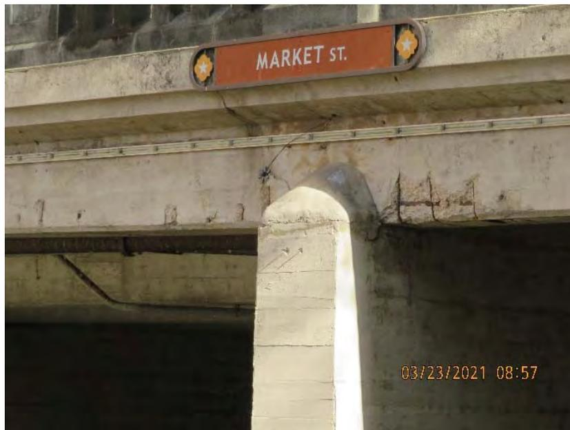
*Figure 6: Typical moderate spalling with exposed reinforcing at exterior south beam*
