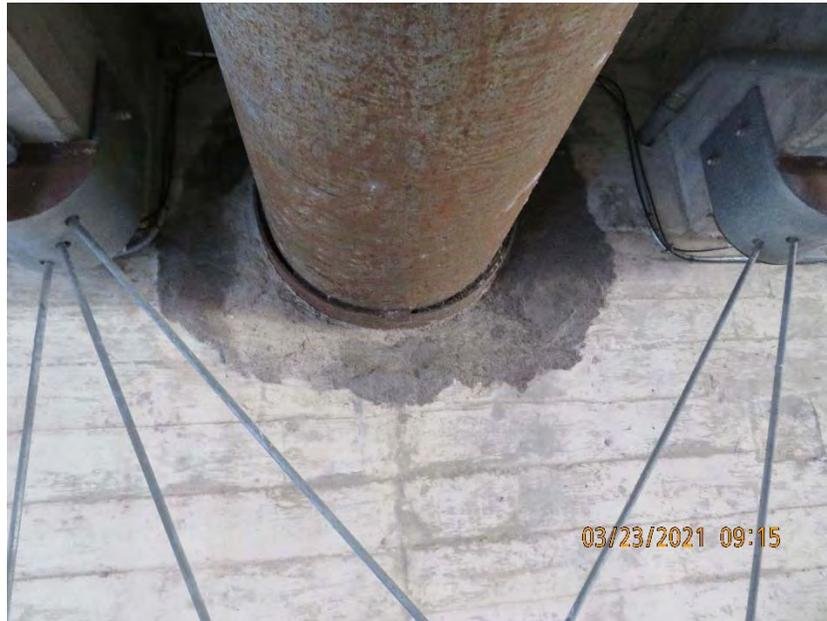
*Figure 2: Patchwork around utility pipe in east abutment wall*
