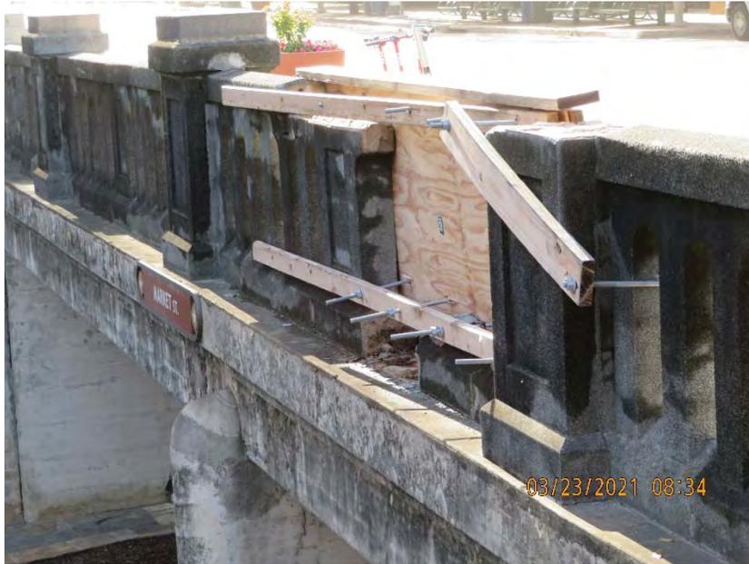
*Figure 18: Major rail damage from vehicular crash*
