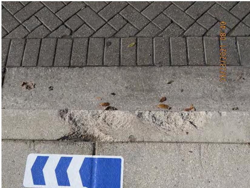
*Figure 17: Minor curb spalling*
