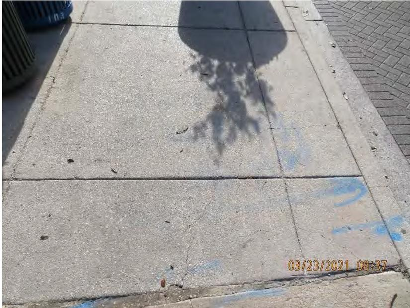
*Figure 16: Typical minor cracking throughout sidewalks*
