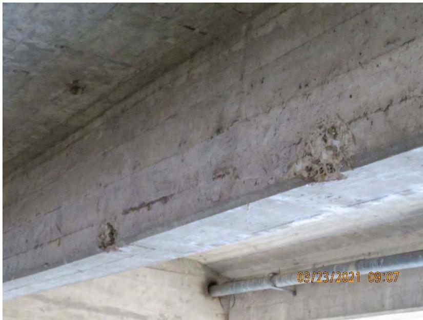
*Figure 9: Typical minor spalling at other interior beams*
