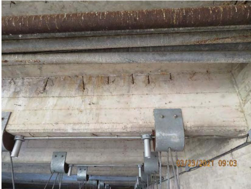
*Figure 8: Moderate spalling with exposed reinforcing at second most southern beam*
