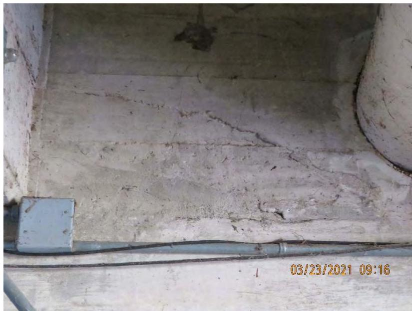
*Figure 1: Minor cracking in east abutment wall*
