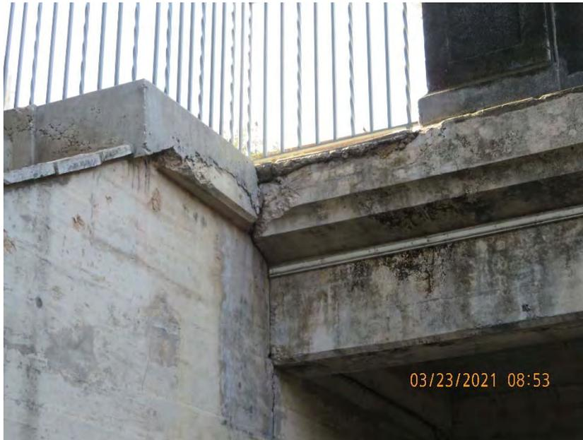
*Figure 10: Major spalling with exposed reinforcing on NE overhang*
