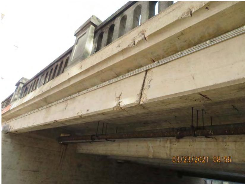
*Figure 11: Typical minor spalling along southern overhang*
