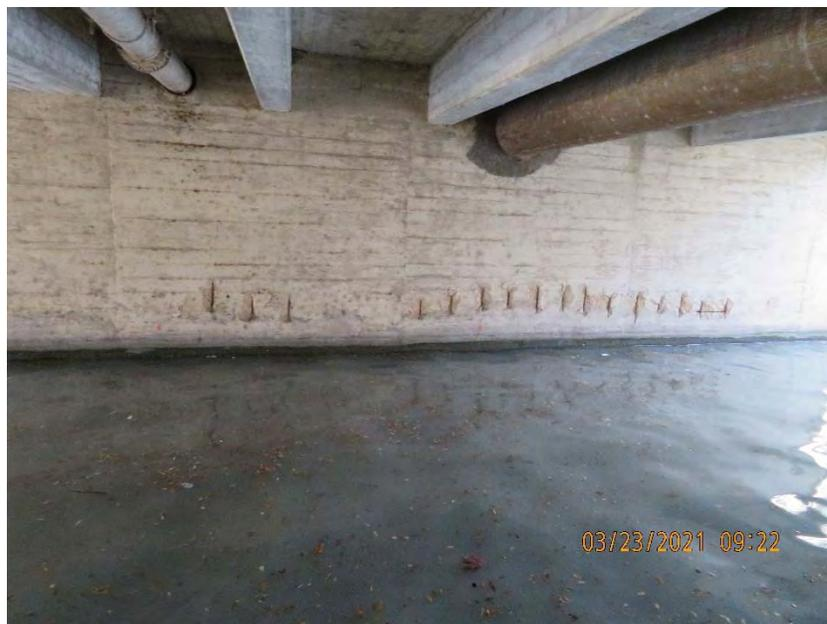
*Figure 3: Moderate spalling with exposed reinforcing at east face of interior bent*
