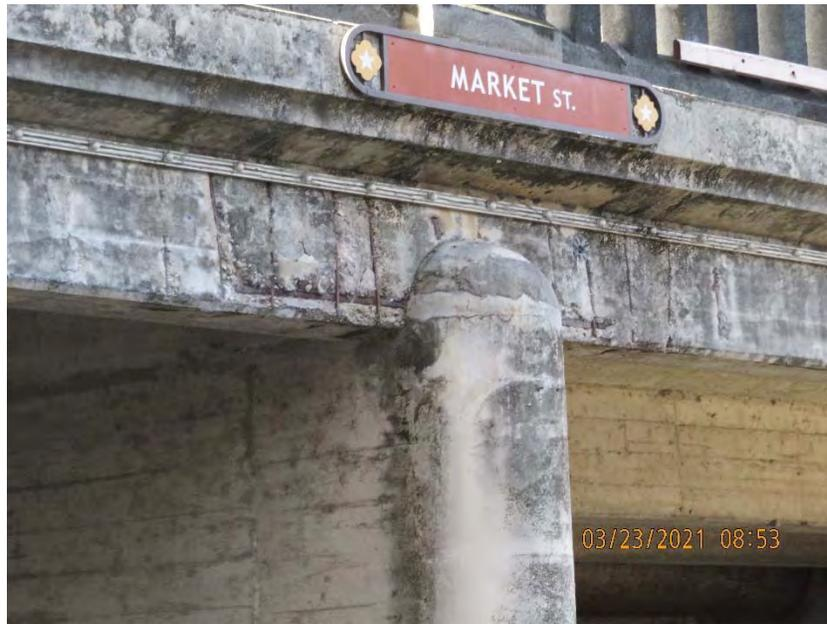
*Figure 4: Typical moderate spalling with exposed reinforcing at exterior north beam*
