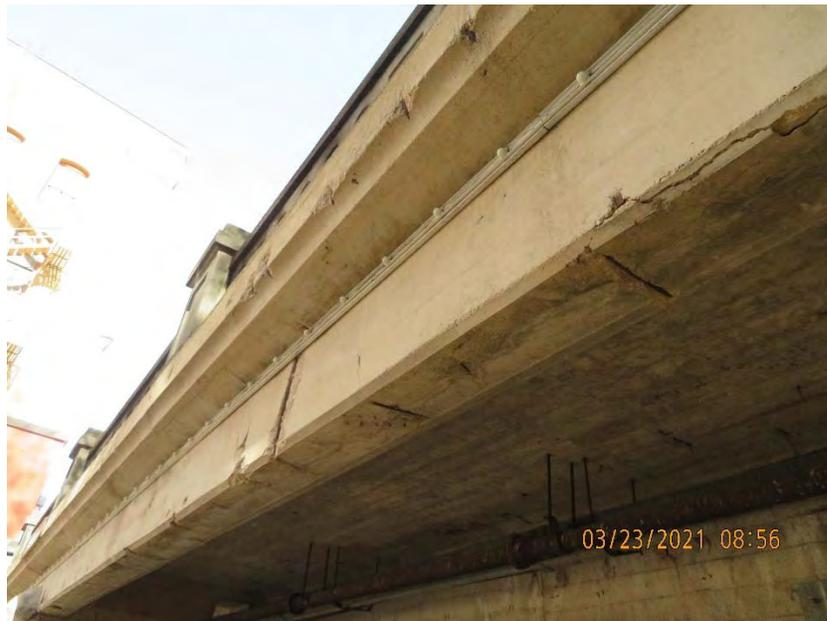
*Figure 7: Moderate spalling & delamination with exposed reinforcing at exterior south beam*
