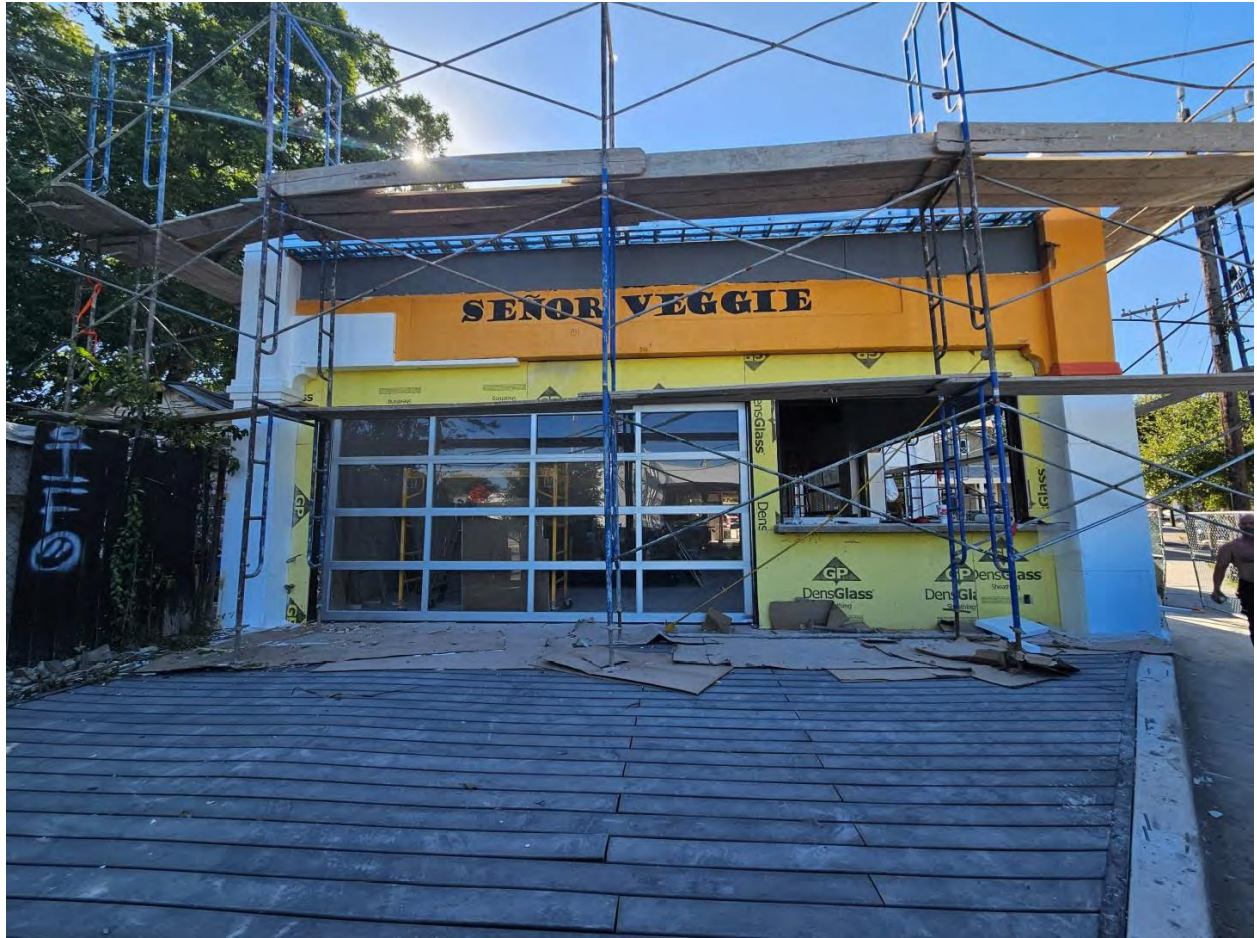
Another photo showing new cladding being installed over the original stucco.
