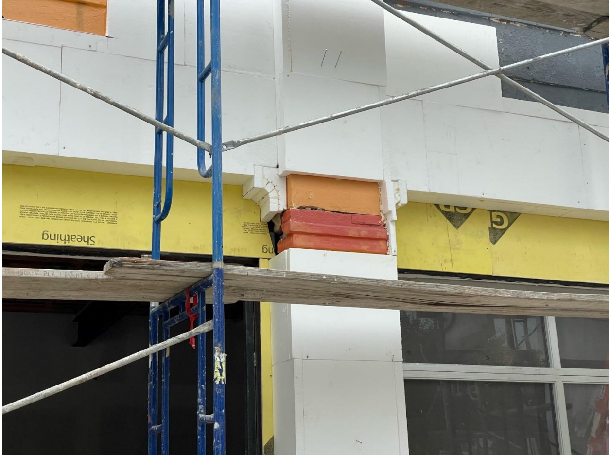
Photo dated 8/22/23 shows increased thickness and revised details at columns.
