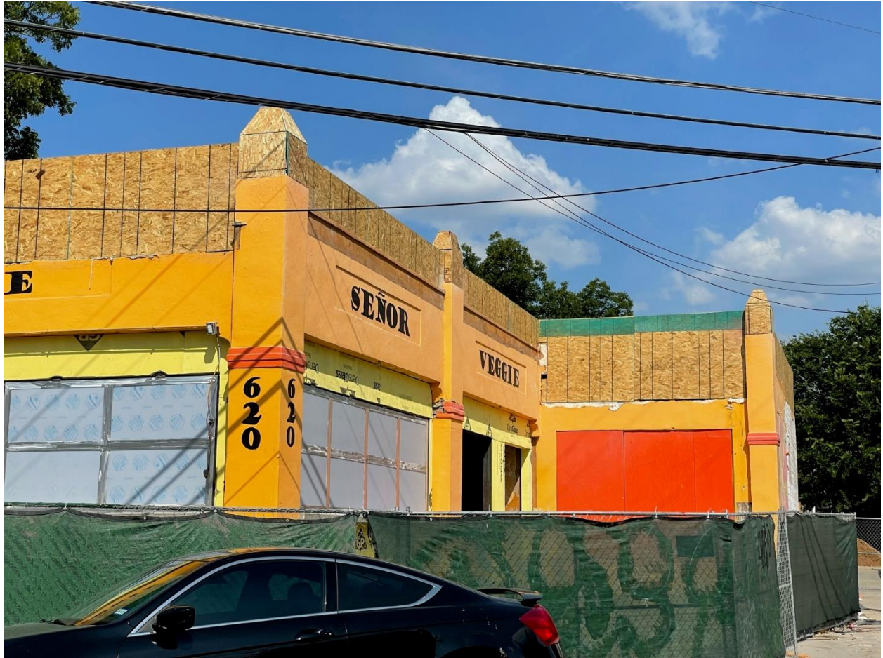
Another photo during construction showing original column conditions. The increase to the parapet height was approved by the HDRC.
