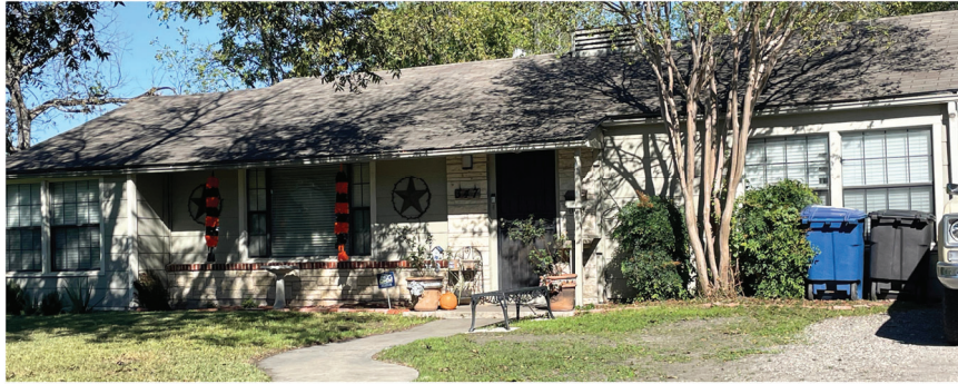
347 Quentin - Wood grain asbestos siding
