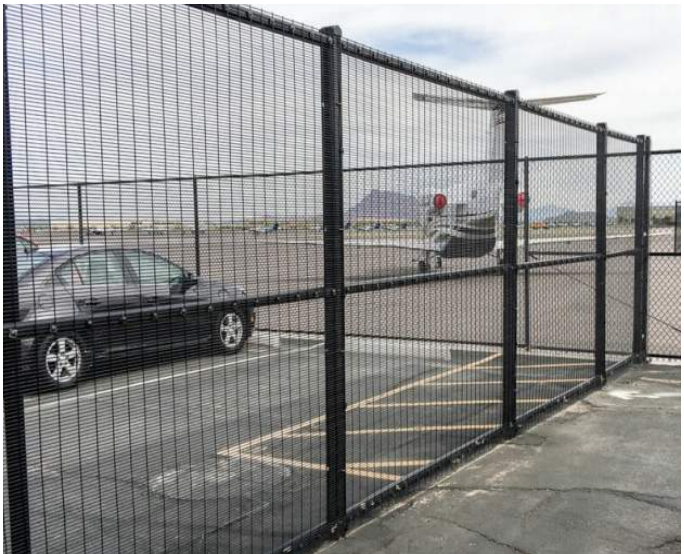
FAA FENCING - ANTI-CLIMB WELDED WIRE FENCE
