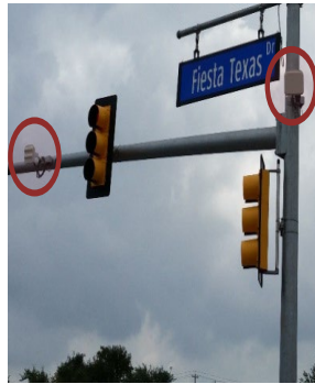
Steel Mast Arms & Vehicle Detection
