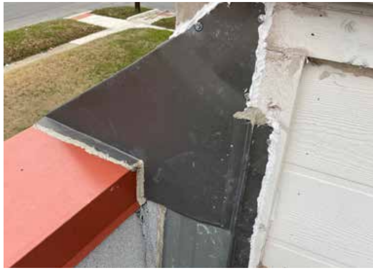
new flashings and sealants applied
