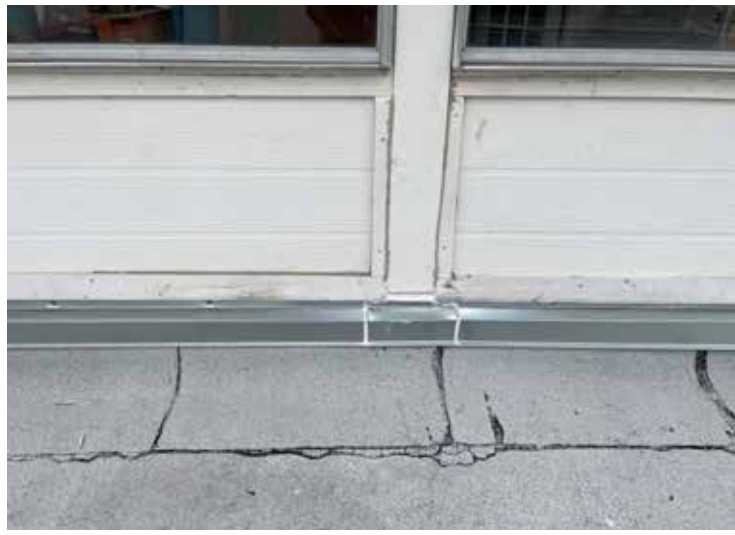
new flashings and sealants applied
