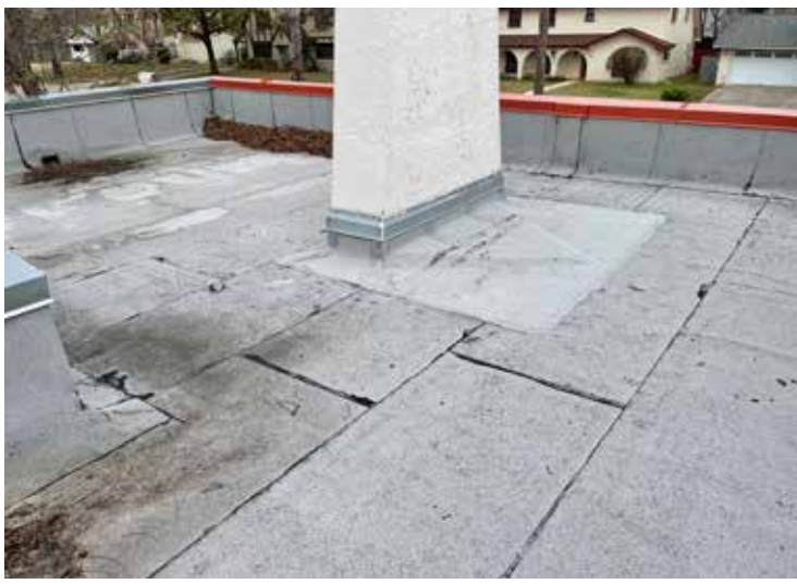
new sbs coating applied
