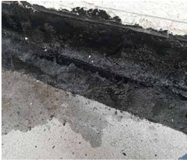
The removed base flashing.
