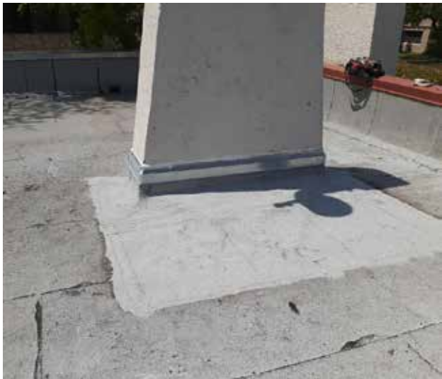
SBS cap sheet installed and metal headwall flashing.
