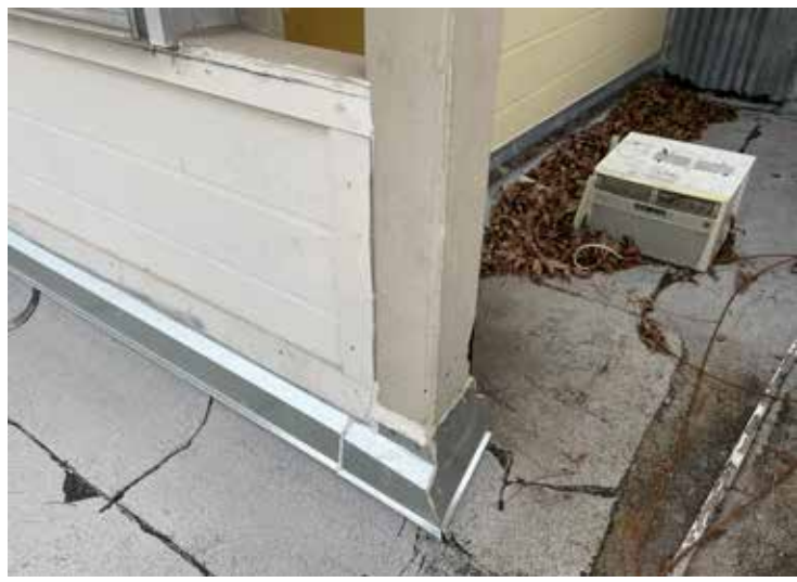
new flashings and sealants applied
