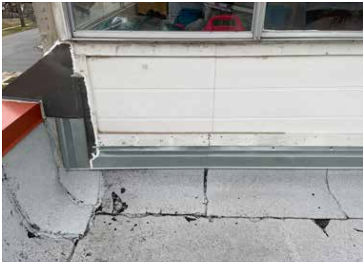
new flashings and sealants applied
