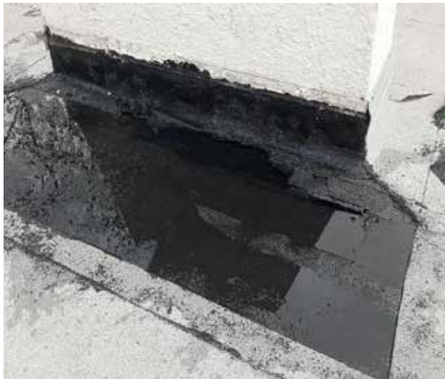
The removed base flashing and area of field.
