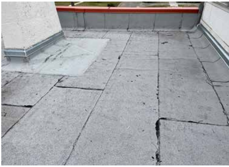
new sbs coating applied
