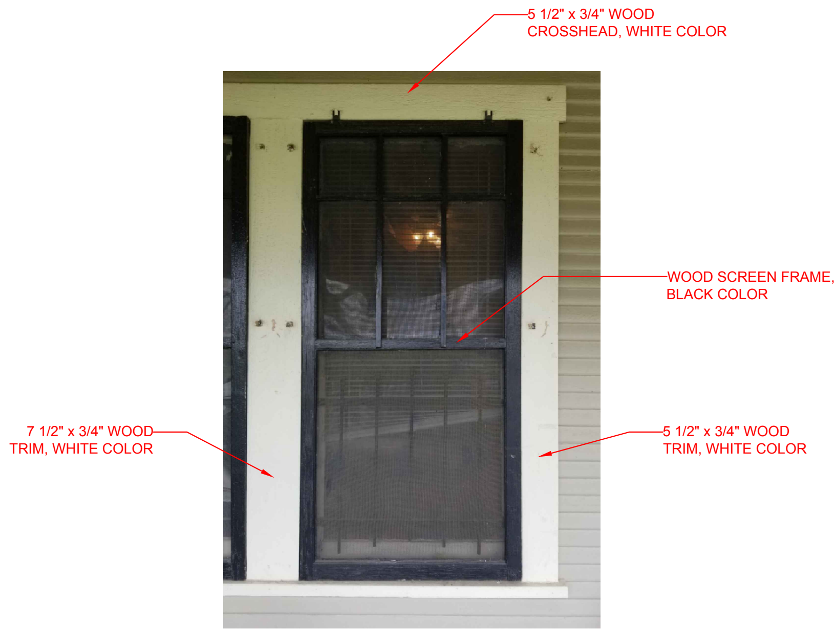
TYP. WINDOW TRIM / SCREEN no scale
