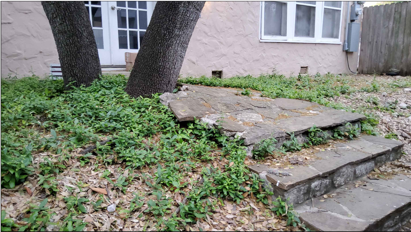
1A L-3C T-5 & T-6 ('LIVE OAKS') LOOKING NORTH-WEST, SHOWING SEVERELY DAMAGED STONE STEP LANDING AREA
