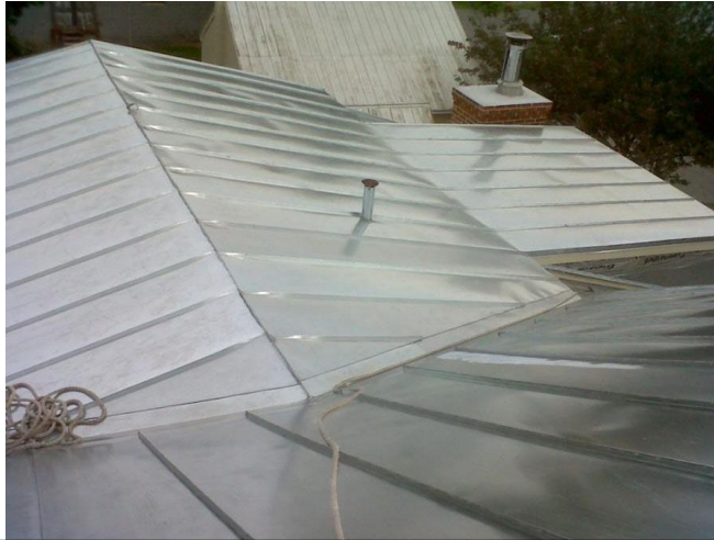
CRIMPED RIDGE STANDING SEAM GALVALUME METAL ROOF
