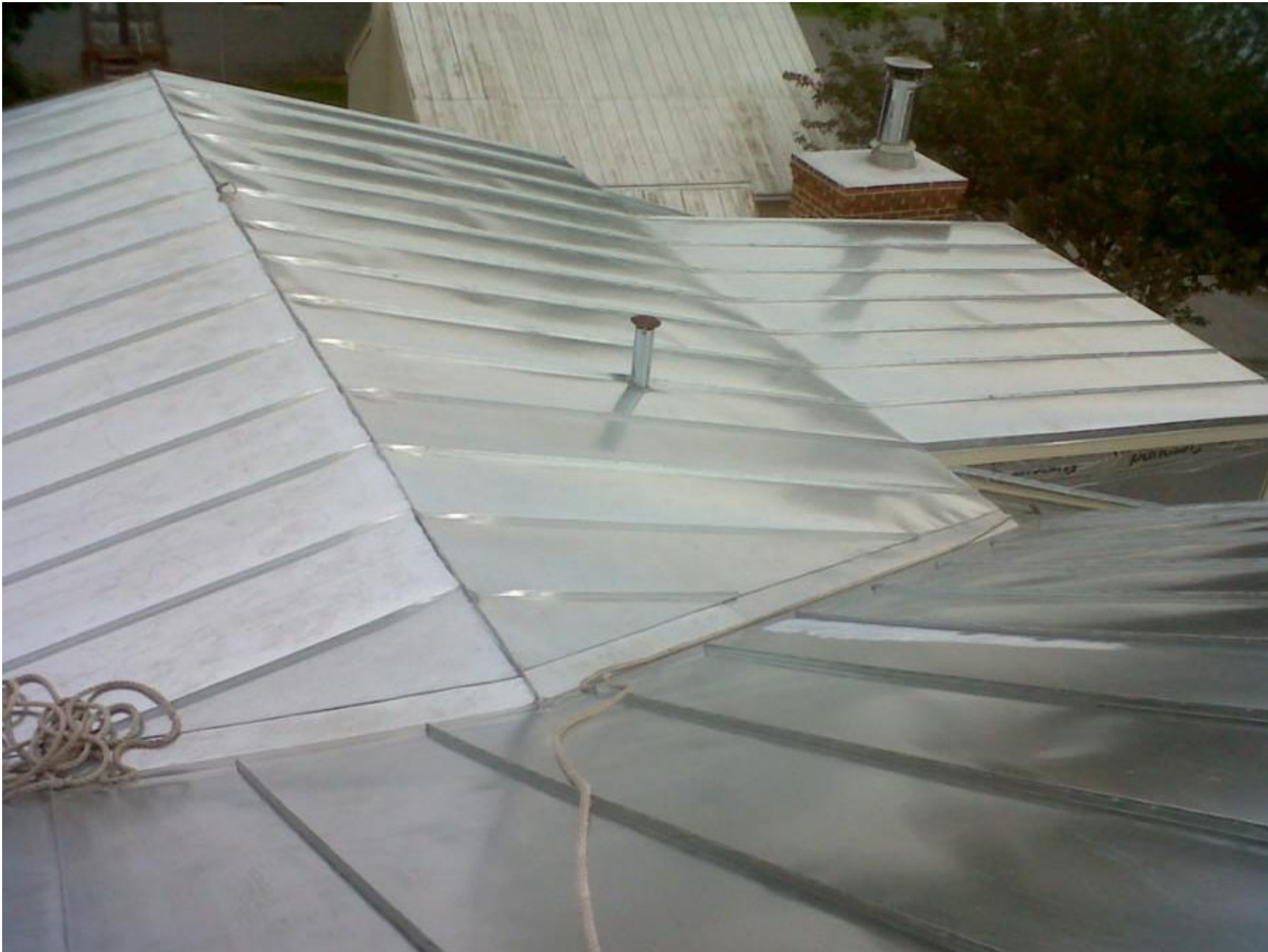
CRIMPED RIDGE STANDING SEAM GALVALUME METAL ROOF
