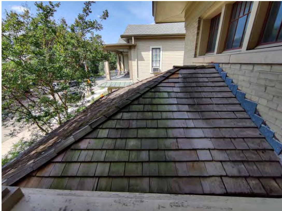
FRONT PORCH WOOD SHINGLE ROOF TO BE REPLACED.
