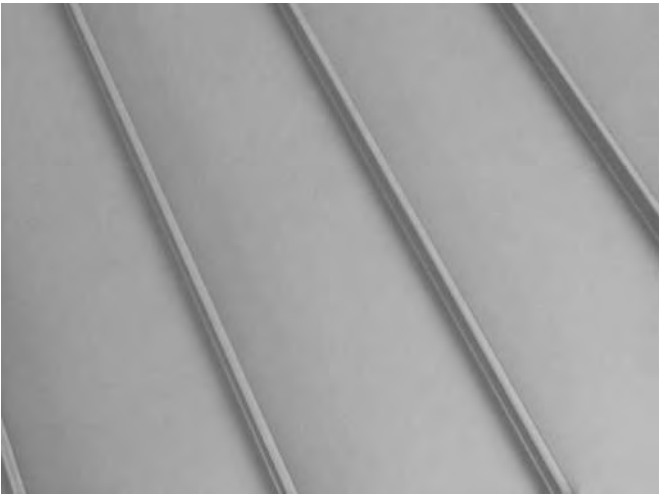
EXISTING GALAVANIZED STANDING SEAM METAL ROOF TO REMAIN
