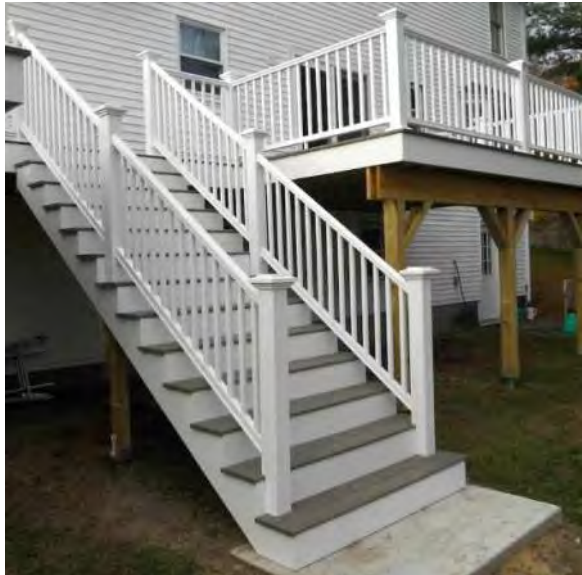
STAIRS WITH COMPOSITE DECK AND RAILING
