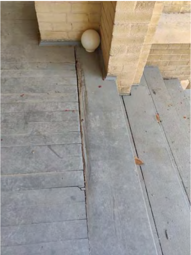
FRONT PORCH WOOD DECK DAMAGE
