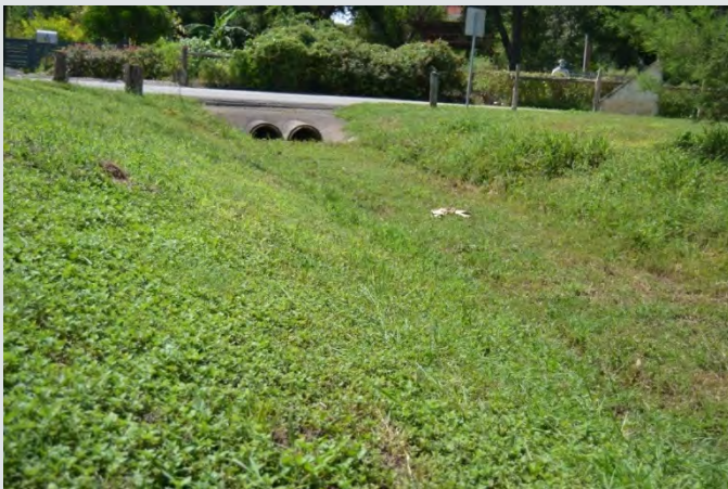
Figure 2.2.5. Example of an earthen swale leading to a concrete culvert that allows two desagues (drainpipes) to allow water to flow beneath the roadway. Source: Photo by HHM, 2021.
