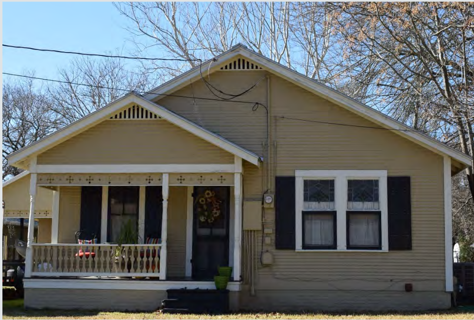
Figure 4.6.2. Example of a porch with a non-original Victorian-inspired “gingerbread” frieze and turned posts and balusters that do not match the period or original style of the house. These elements create a false historic appearance. Removal of the brackets is recommended but not required. Source: Photo by HHM, 2020.
