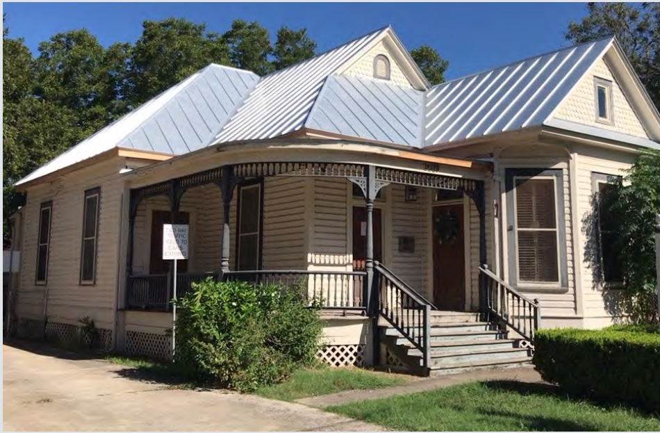
Figure 4.5.2. Example of a metal roof on a historic bungalow. Metal roofing is only appropriate throughout the district, provided that its installation does not remove or damage character-defining historic features. For buildings dating before 1945—like this one—the ridge cap and seams for the metal roof are recommended to comply with the “Checklist for Metal Roofs” in the citywide guidelines. Source: Photo by OHP, 2022.
