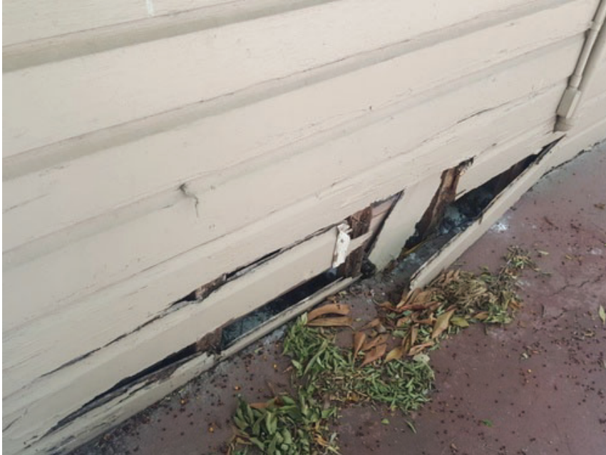
Wood rot to include studs and siding
