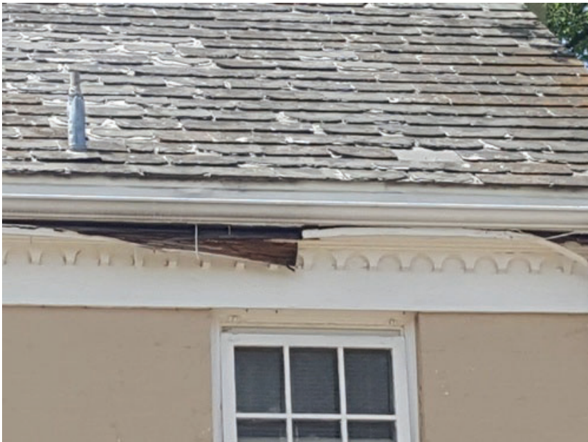
Carpentry damage as well as shingle damage
