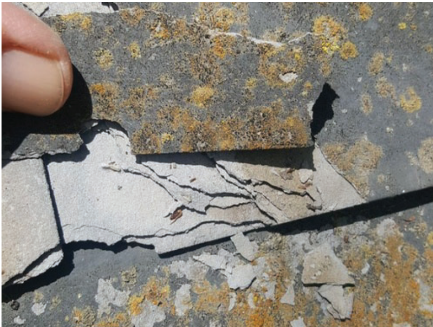
Asbestos shingles installed prior to 1977
