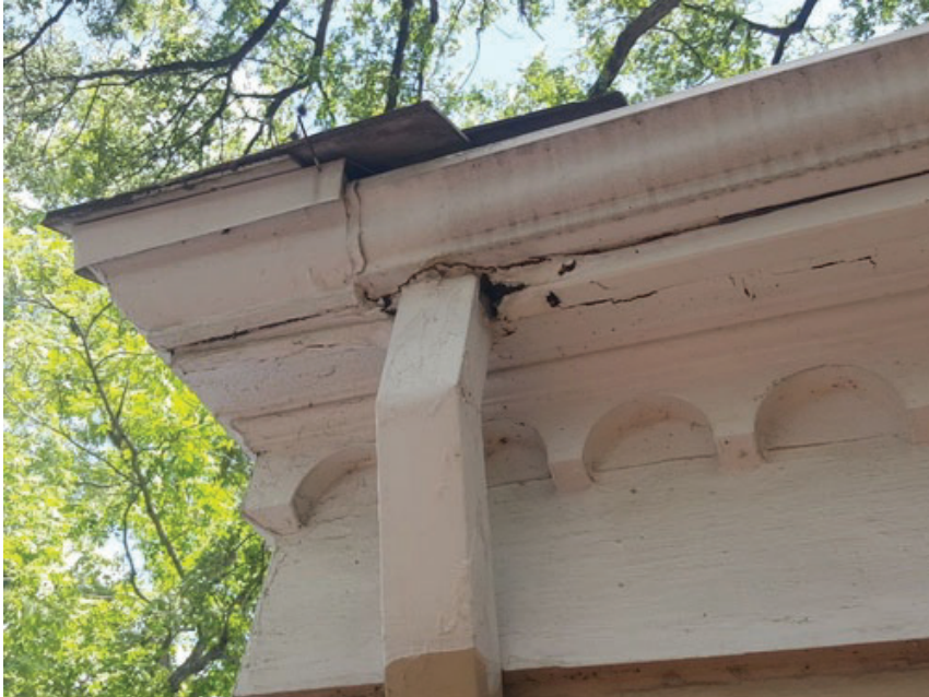
Uneven gutters are clogged
