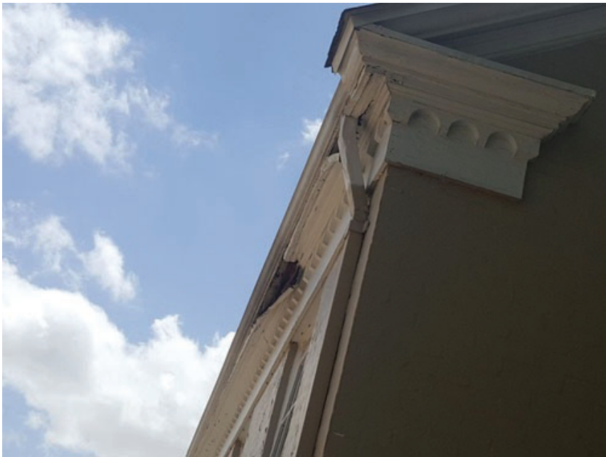
Soffit and fascia damage to be done prior to roof replacement
