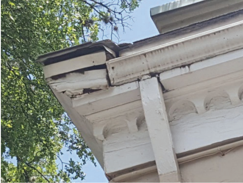
Uneven damming causing more damage
