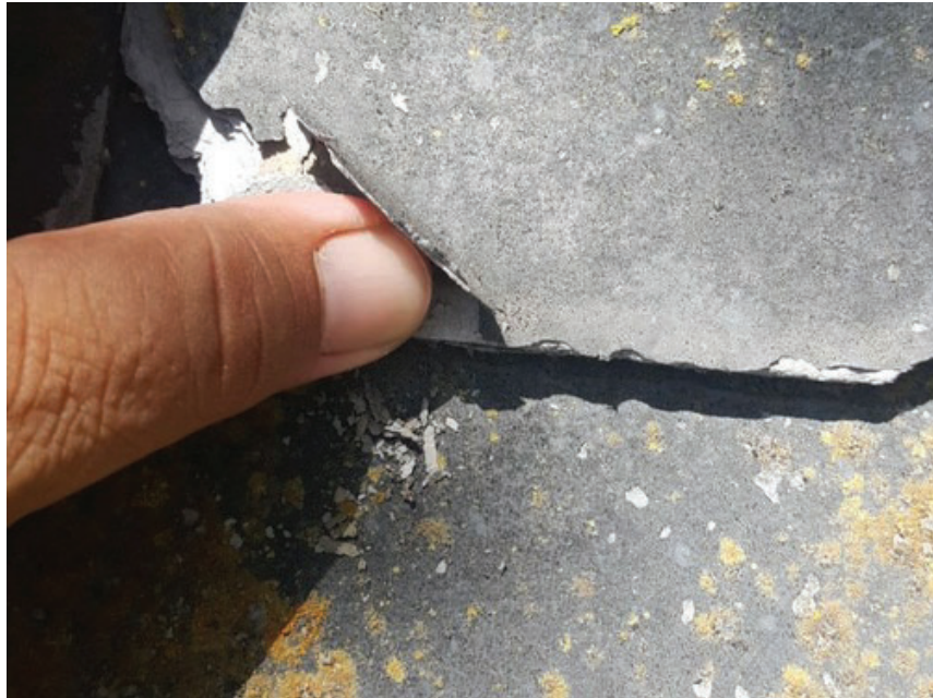
Flaking shingles starting to breakdown
