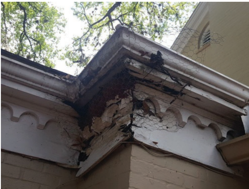
Repairs to be done prior to roof Previous repairs with chicken wire to prevent rodent intrusion
