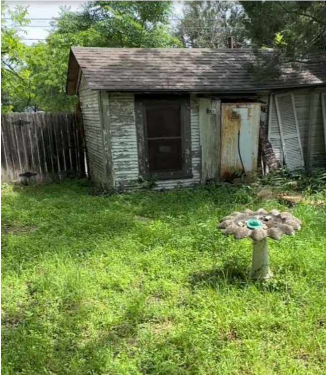
319 W LULLWOOD ST. ACCESSORY UNITS BUILD AROUND 1926, NO FOUNDATION PRESENT
