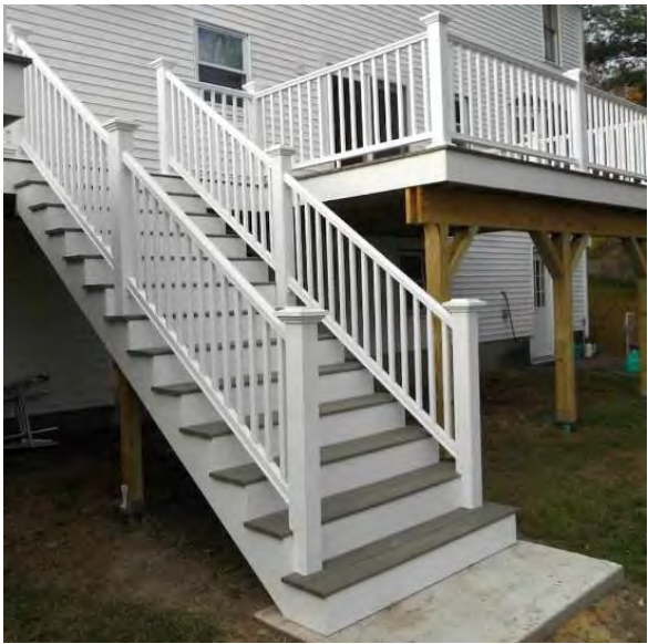
STAIRS WITH COMPOSITE DECK AND RAILING
