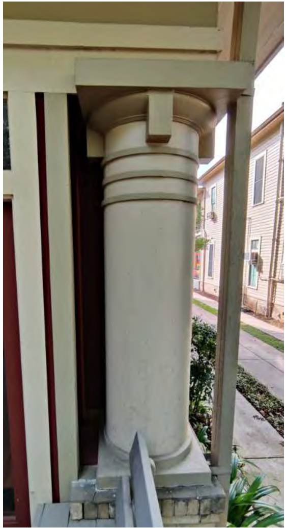
NEW PORCH COLUMN AND BRICK PILASTER TO MATCH EXSTING DETAILING
