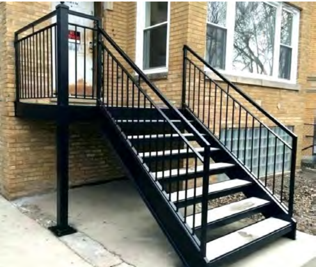
PAINTED STEEL STAIRCASE AND RAILING
