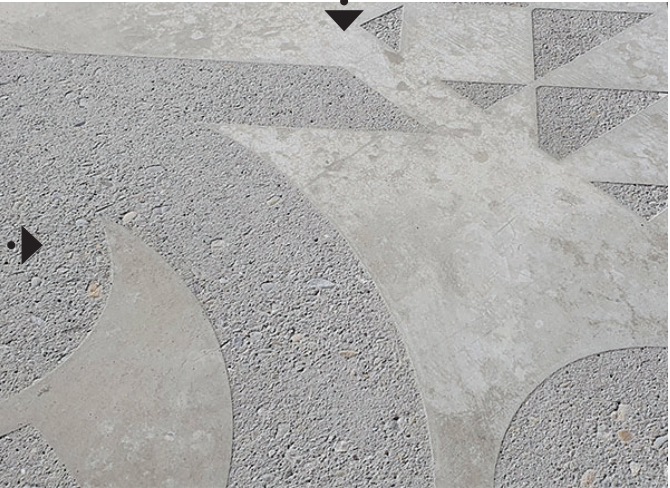
PROPOSED Flooring: SANDBLASTED concrete with R. Burle Marx inspired design
