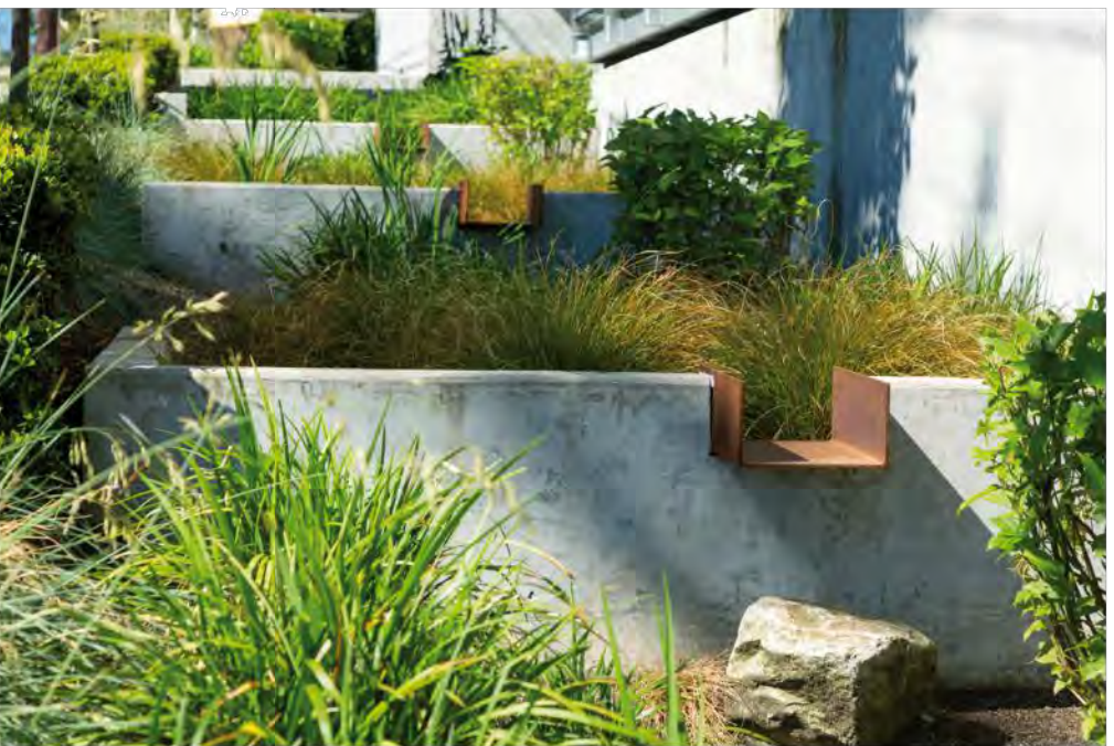
TERRACED WALLS AND SCUPPERS DIRECT SURFACE RUNOFF FROM MYRTLE STREET INTO A LID DETENTION BASIN. WATER TO BE FILTERED BY SOIL PROFILE BEFORE BEING DISCHARGED INTO THE SAN ANTONIO RIVER.
