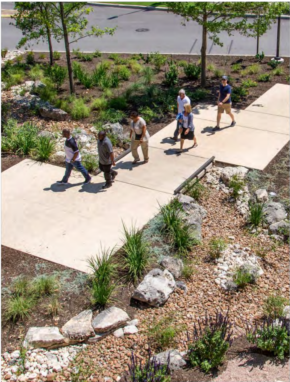
GRAVEL SWALE TO DIRECT SURFACE RUNOFF AND MULTIFAMILY RAINWATER AND BUILDING CONDENSATE INTO LID INLET. LANDSCAPE BOULDERS TO BE PLACED AROUND THE GRAVEL SWALE, LID DETENTION BASIN, AND IN OTHER KEY AREAS IN THE LANDSCAPE.
