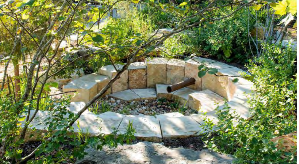
LID INLET TO FUNNEL WATER INTO UNDERGROUND STORAGE TANK WITH SAND FILTER. RECLAIMED WATER TO POTENTIALLY BE USED FOR IRRIGATION.
