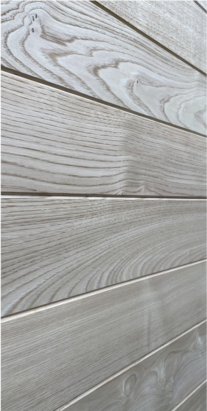
Close-up of ash siding in C-20 profile by Thermory.
