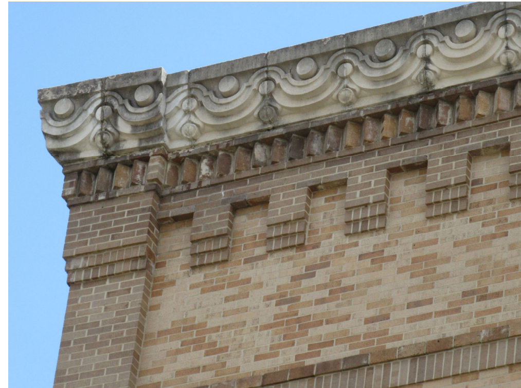
Recreated/Relocated Masonry at Crown
