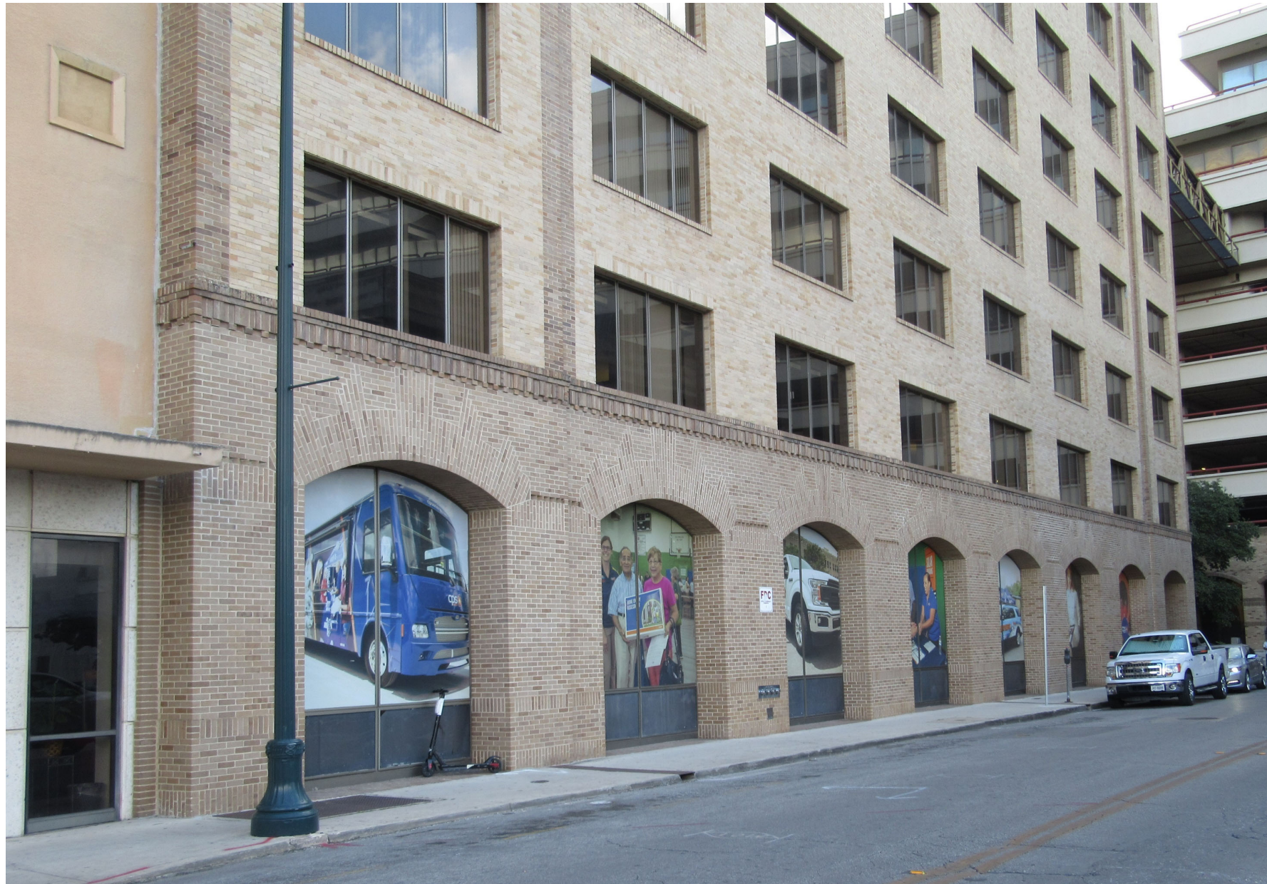
Reinstated Masonry Arches
