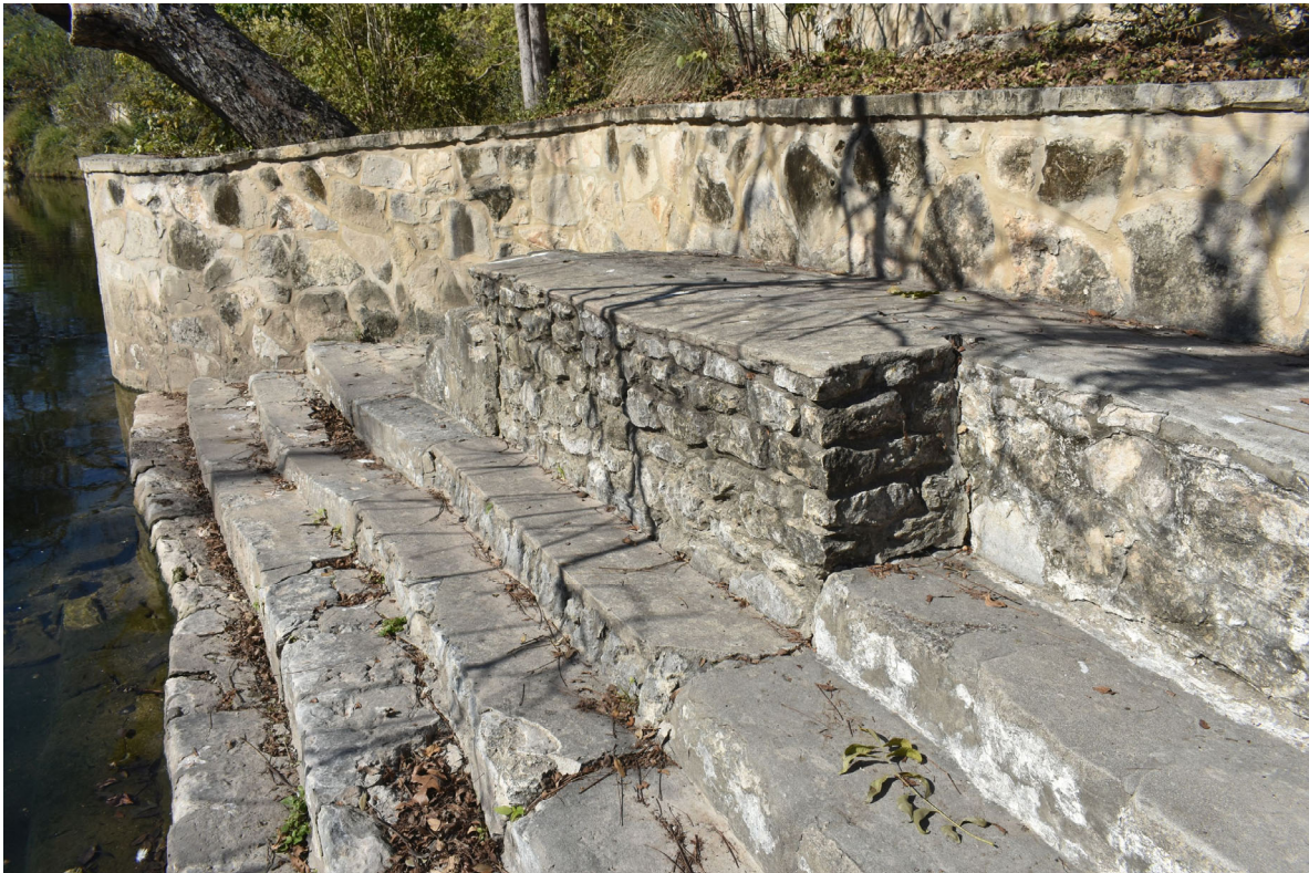
Detail of stone rubble platform addition (D) and modified wall (E); view facing northwest
