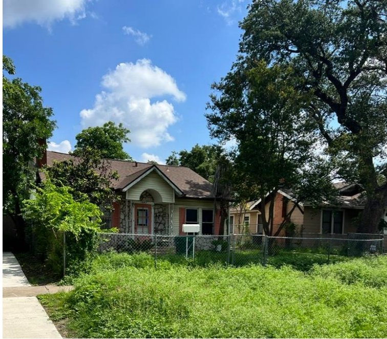
Neighboring property view to west
