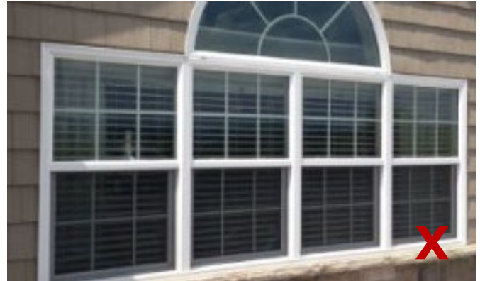
Windows that are not consistent with the Guidelines negatively impact a project's ability to appear compatible within a historic district.
