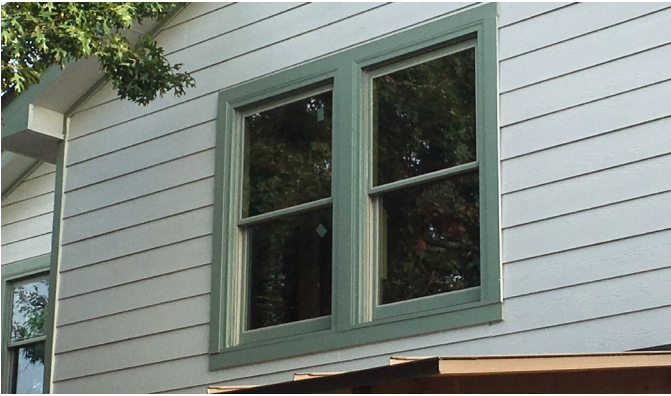
These windows feature a traditional profile, installation depth, and proportions that are consistent with the Guidelines.
