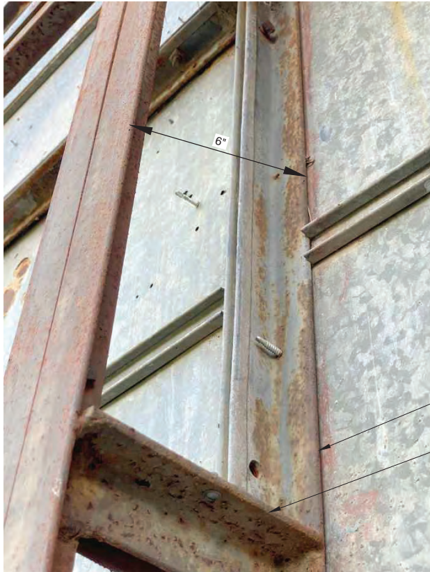
1 QUAD ANGLE FRAME MEMBER NOT TO SCALE
