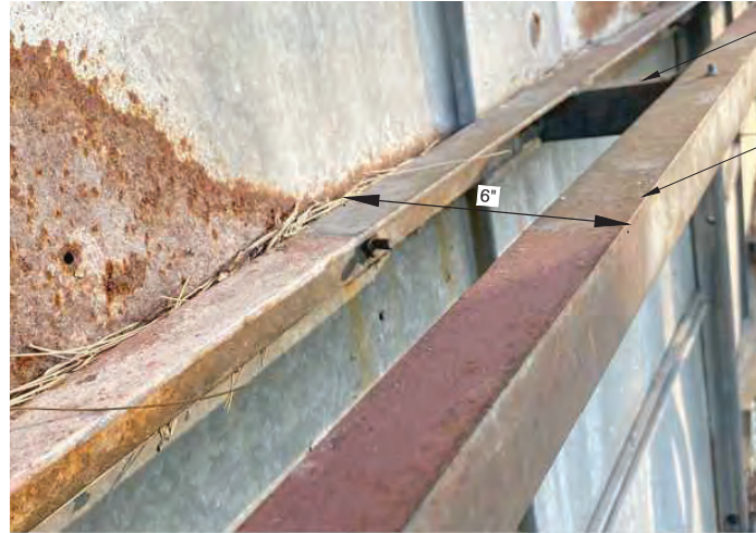
2 DOUBLE ANGLE FRAME MEMBER NOT TO SCALE
