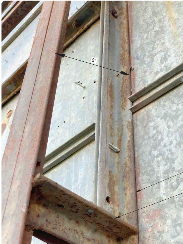
1 QUAD ANGLE FRAME MEMBER NOT TO SCALE
