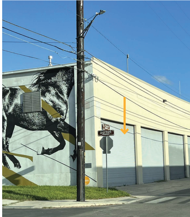
225 n swiss st - corrugated metal siding
