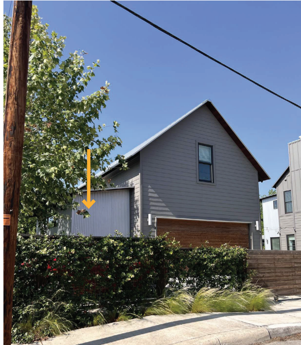
1103 pine st - galvalume corrugated metal siding, dark gray painted siding
