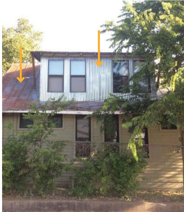
rusted metal roof, corrugated siding
