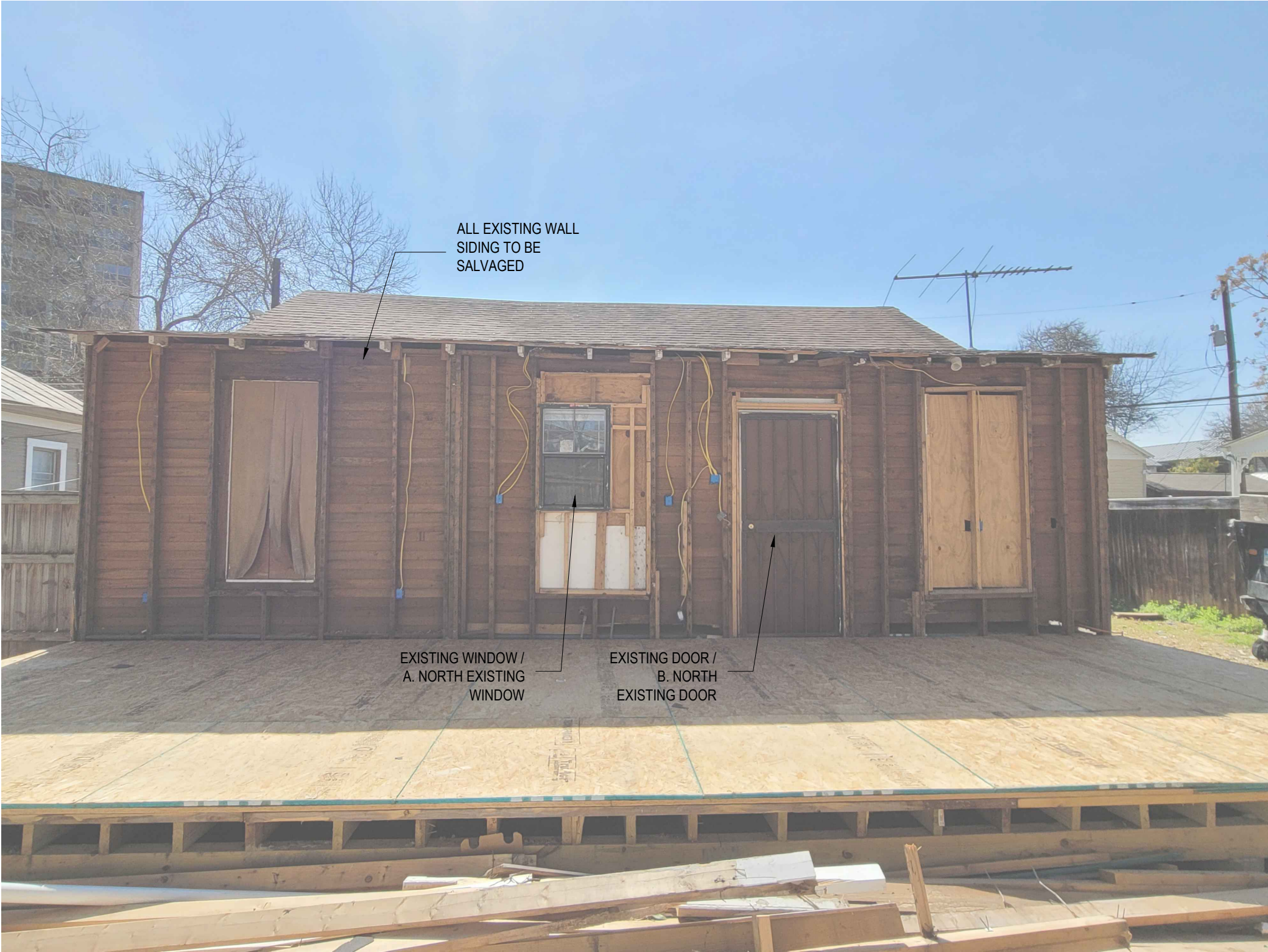
4 NORTH EXISTING ELEVATION 1/4" = 1'-0"
