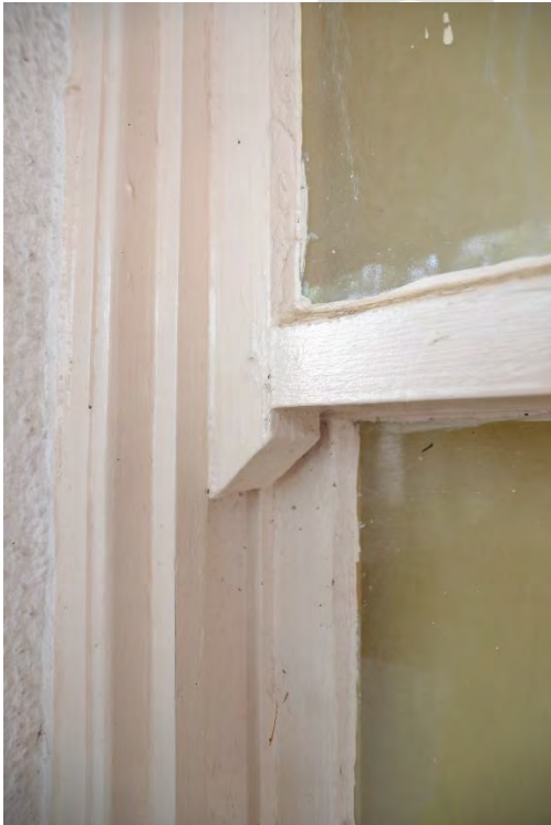
Figure 5. Upper sash tail block detail on an original window. Sash contains glazing putty. Sash is painted shut.
