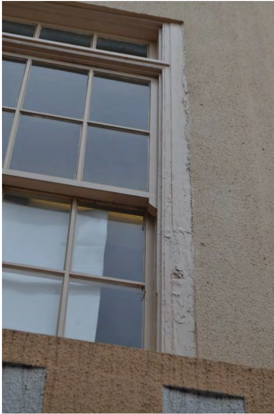
Figure 11. Damage to frame at west stair window.
