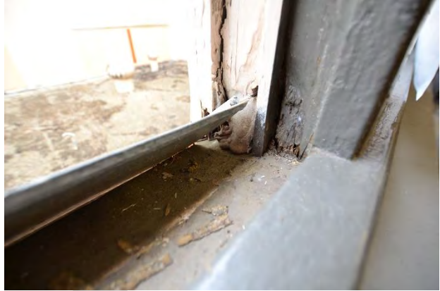
Figure 16. Rotted frame and inappropriate sealant repair at window jamb and sill. Moisture damage likely exacerbated by loose-laid sill pan flashing.
