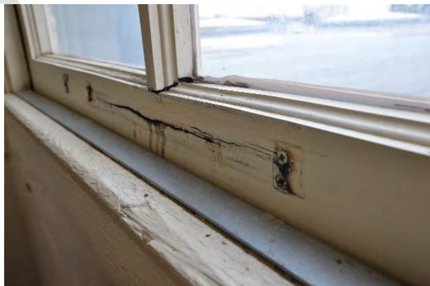
Figure 14. Roof flashing tied into windowsill.
