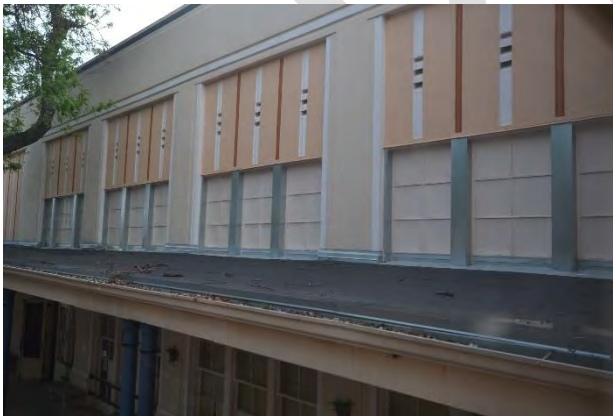
Figure 9. West elevation auditorium windows have been blocked off.
