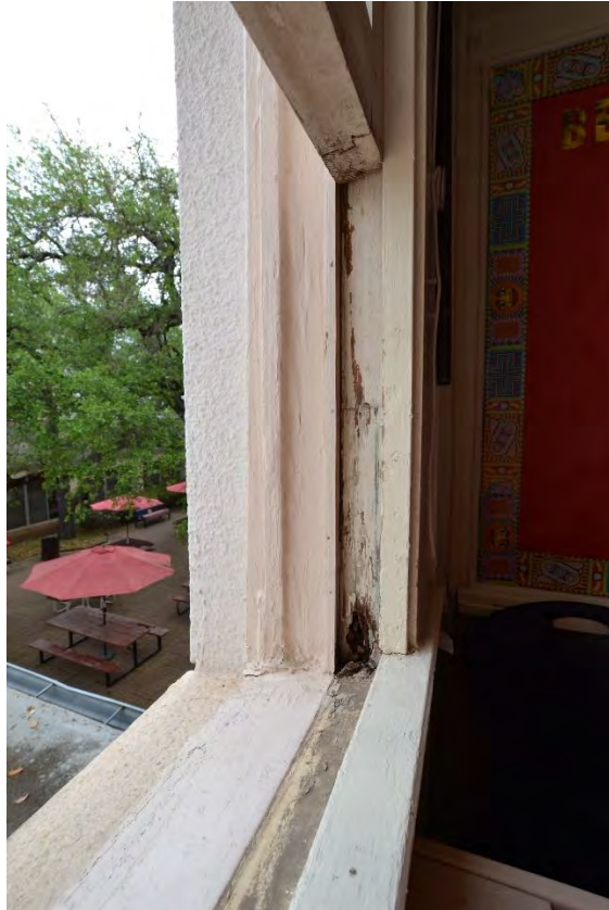
Figure 12. Rotted frame at window jamb and sill.
