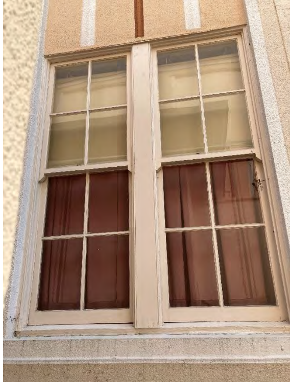
Figure 4. Replacement double hung sashes in an original frame, east elevation of auditorium.
