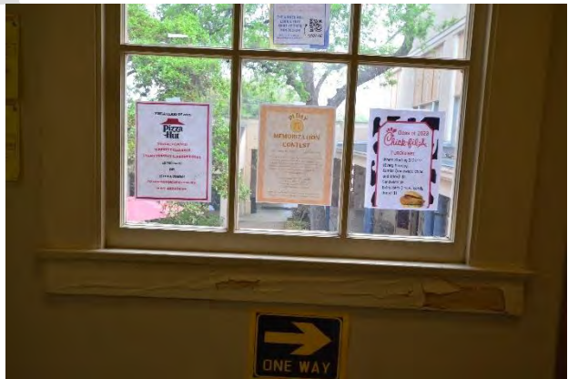
Figure 10. Moisture damage at the apron, sill and adjacent wall in the east stair.
