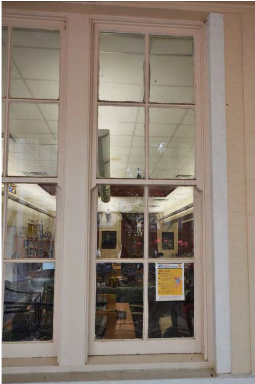
Figure 3. Original double hung sashes in an original frame, east elevation of library in courtyard.
