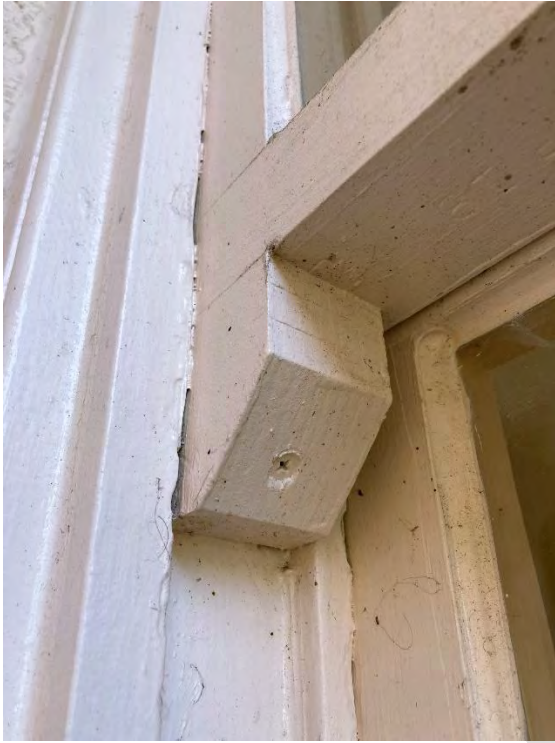
Figure 7. Upper sash tail block detail on a replacement window with sealant at glazing. Sash is screwed in place.
