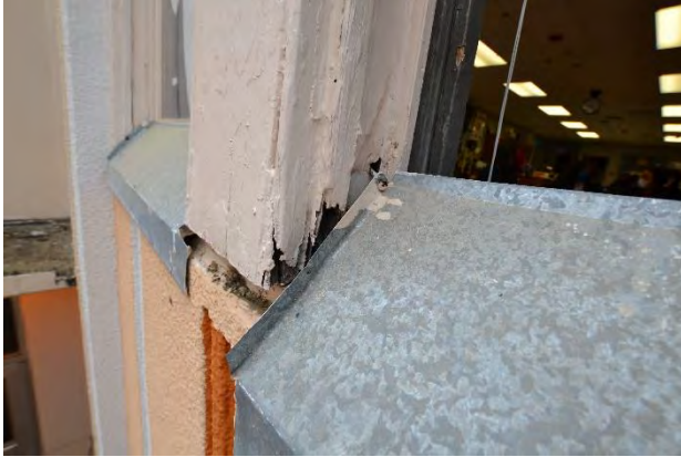
Figure 15. Moisture damage at stile and loose-laid sill pan flashing.
