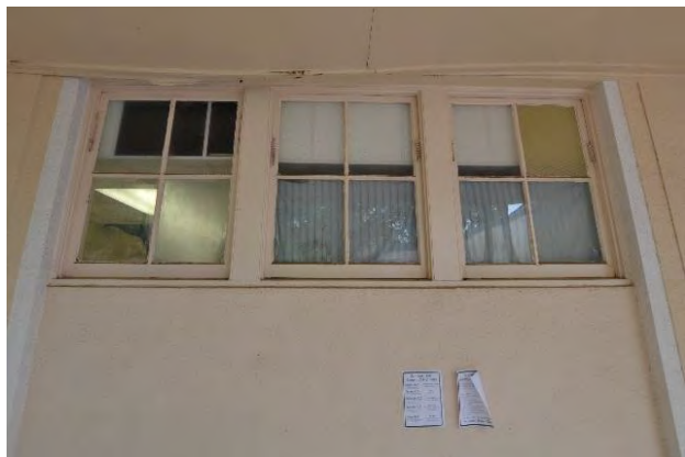
Figure 20. Mismatched replacement glazing.
