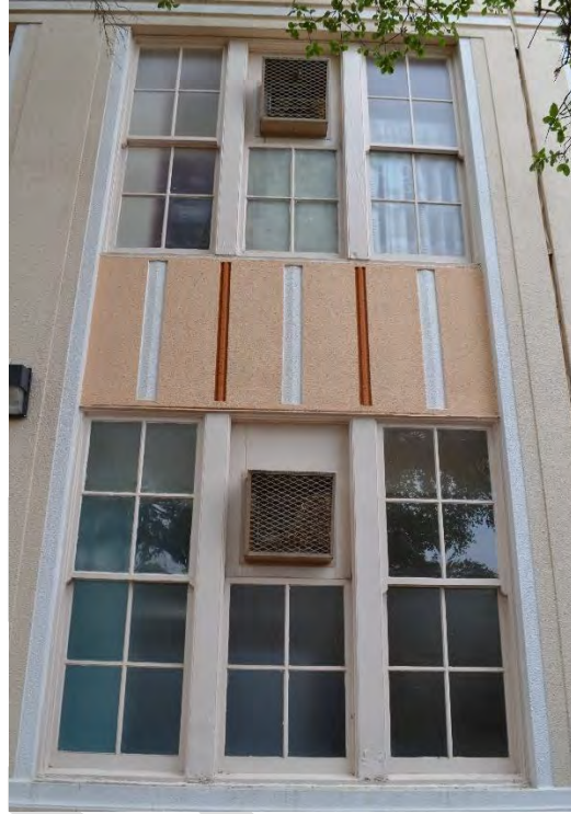
Figure 8. Removed sashes and inappropriate repairs at stiles.
