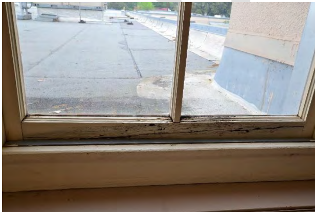
Figure 13. Moisture damage at sash near plane of roof. Note roof flashing turned into frame at sill.
