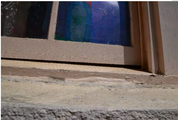
Figure 17. Window not fully closed.
