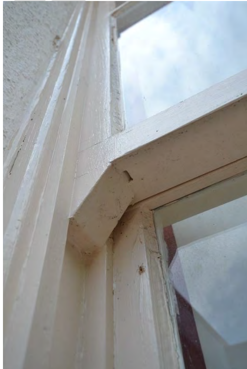
Figure 6. Upper sash tail block detail on a replacement window with sealant at glazing. Sash is painted shut.
