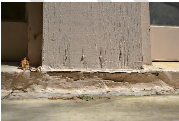
Figure 19. Deterioration at mullion and sill.
