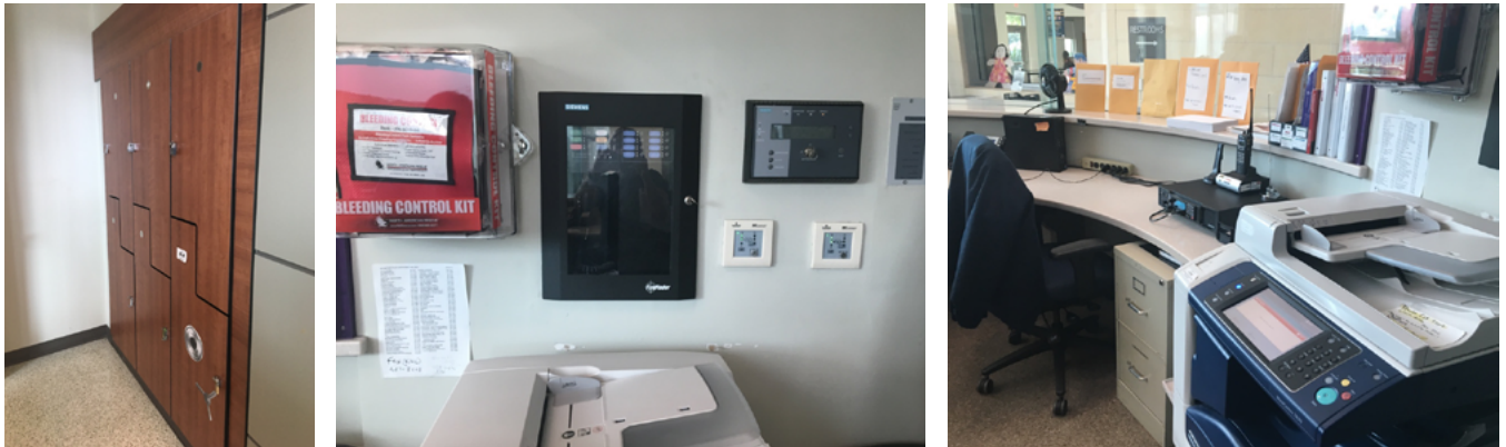
Service Agent Lockers, Blood Control, Fire Control Panel, Copier, Radio
