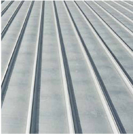
STANDING SEAM METAL ROOF FEATURE SMOOTH PANELS MEASURING 18 TO 21 INCHES IN WIDTH, A STANDARD GALVALUME FINISH, AND A CRIMPED OR MUNCH RIDGE SEAM.
