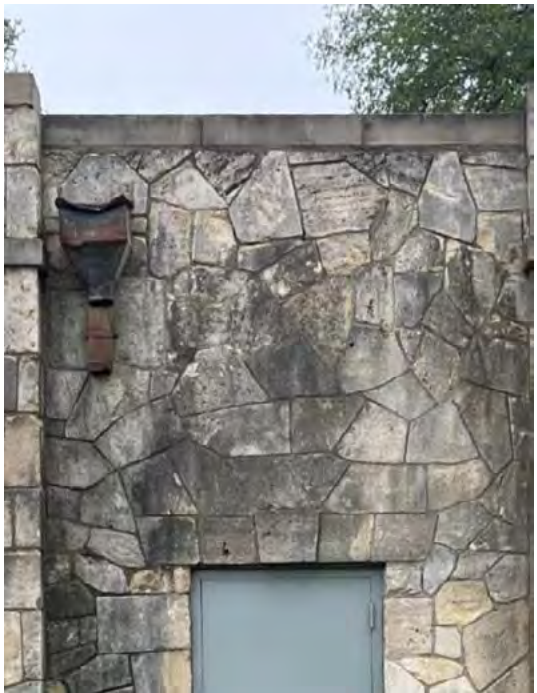
Clean stonework, remove rusted scupper box and downspout, re-point mortar joints & patch stone at scupper opening.
