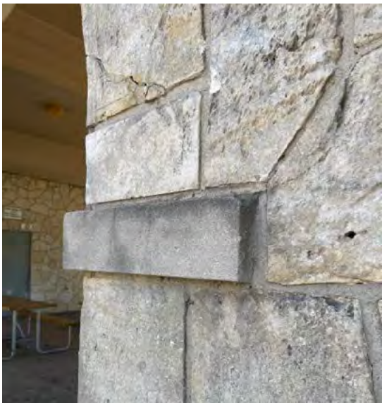
Repair and clean damaged cast stone bands.
