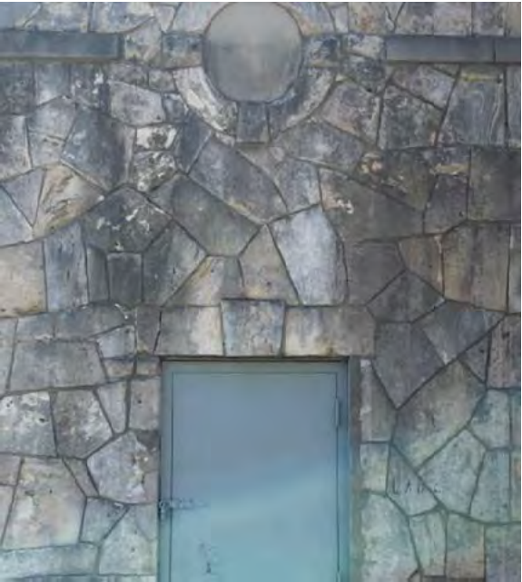
Clean stonework typ. Re-point mortar joints. Re-open (2) circular ventway and install new wood grille and mesh backer.
