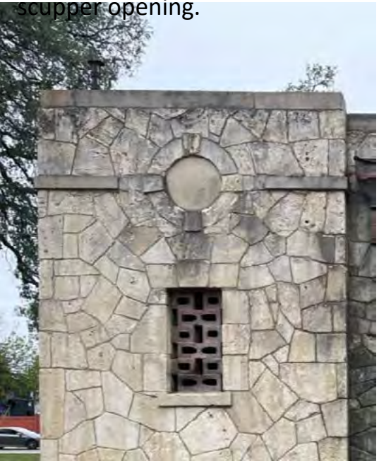
Clean stonework typ. Re-point mortar joints. Re-open circular ventway and install new wood vent cover. Patch cast stone banding above window opening.
