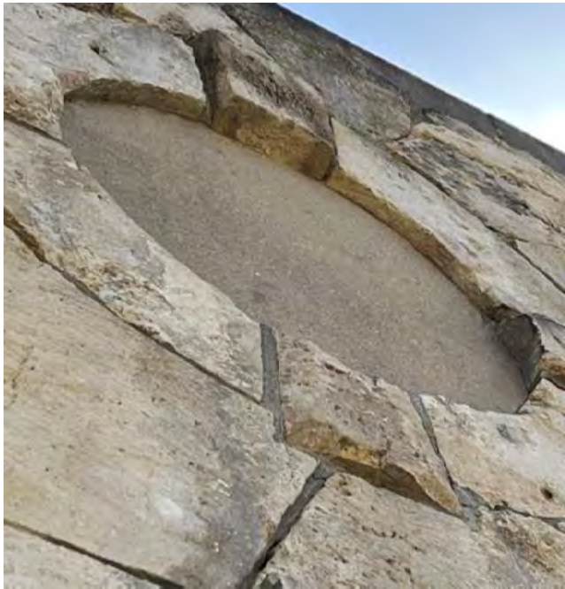
Re-open (1) circular ventway and install new wood grille and mesh backer.
