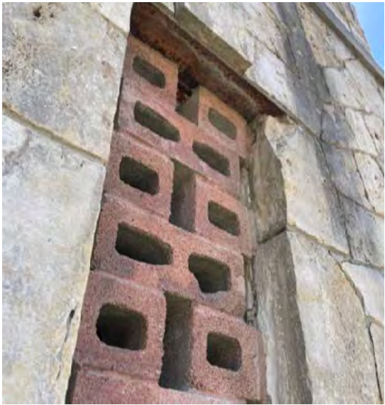
Remove CMU screen and rusted steel lintel, replace with new terracotta breeze block infill and steel lintel.
