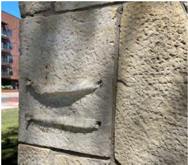
Repair pits and cavities on stone arch (typical condition).
