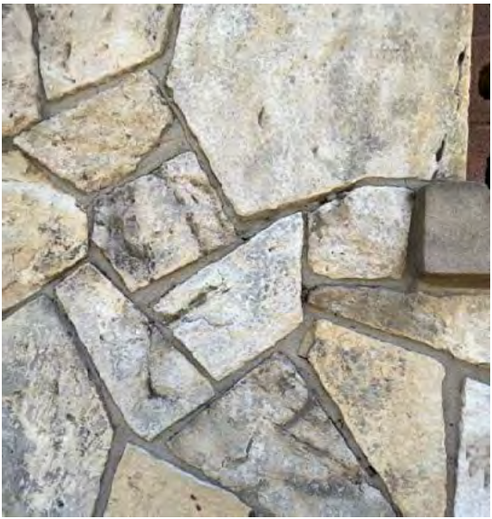
Clean stonework, re-point mortar joints.
