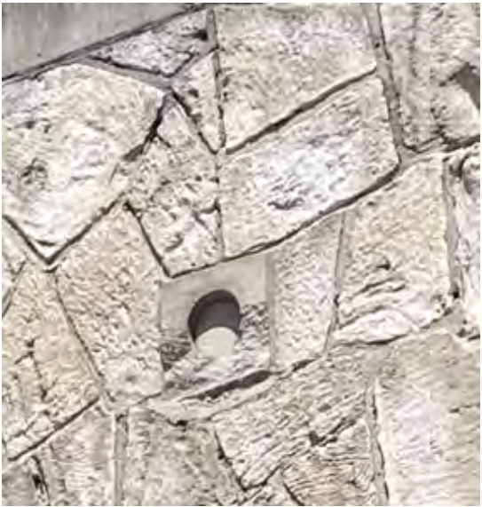
(2) canales scuppers missing and capped, needs repair, re-open, re-point mortar joints.
