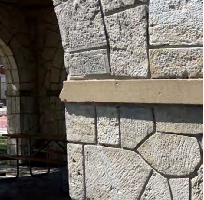
Repair cast stone bands where eroded or damaged.
