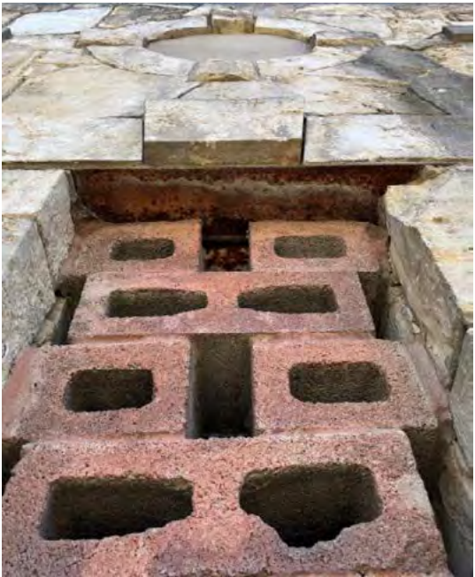
Remove CMU screen and rusted steel lintel, replace with new terra cotta breeze block infill and steel lintel.
