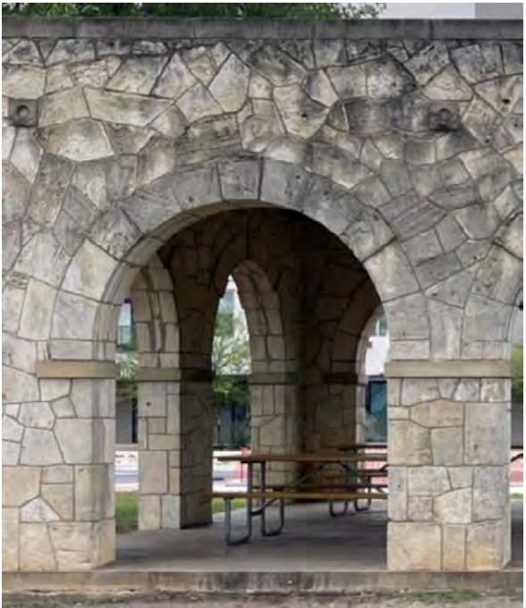
Clean stonework, (3) canales scuppers missing and capped, needs repair, re-open, re-point mortar joints.
