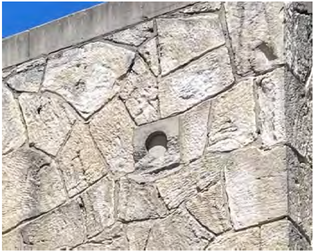
(1) canale scupper missing and capped, needs repair, re-open, re-pointing joints and fill in cavities on stone.
