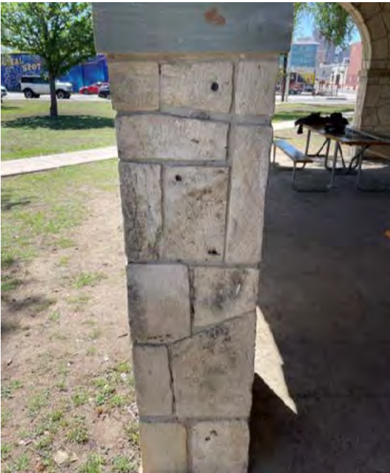
Clean stonework typ. Re-point mortar joints. Rust deposits left from previous iron gates (typical inside archways).
