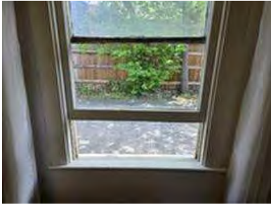
Location: Bedroom 2 Notes: Rotting frame, missing apron
