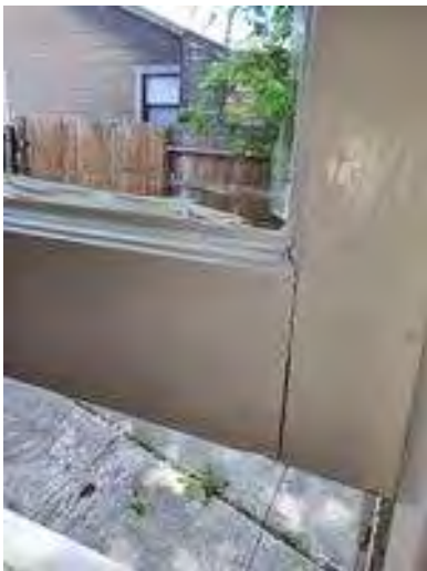
Location: Bedroom 2 Notes: -Cracked frame -Water damage
