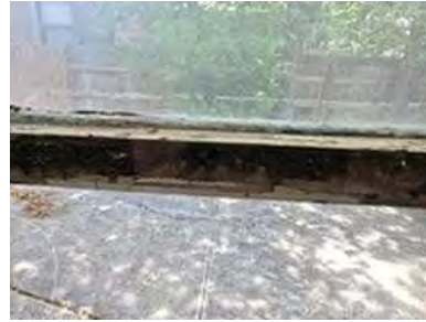
Location: Bedroom 2 Notes: water damage, wood rot
