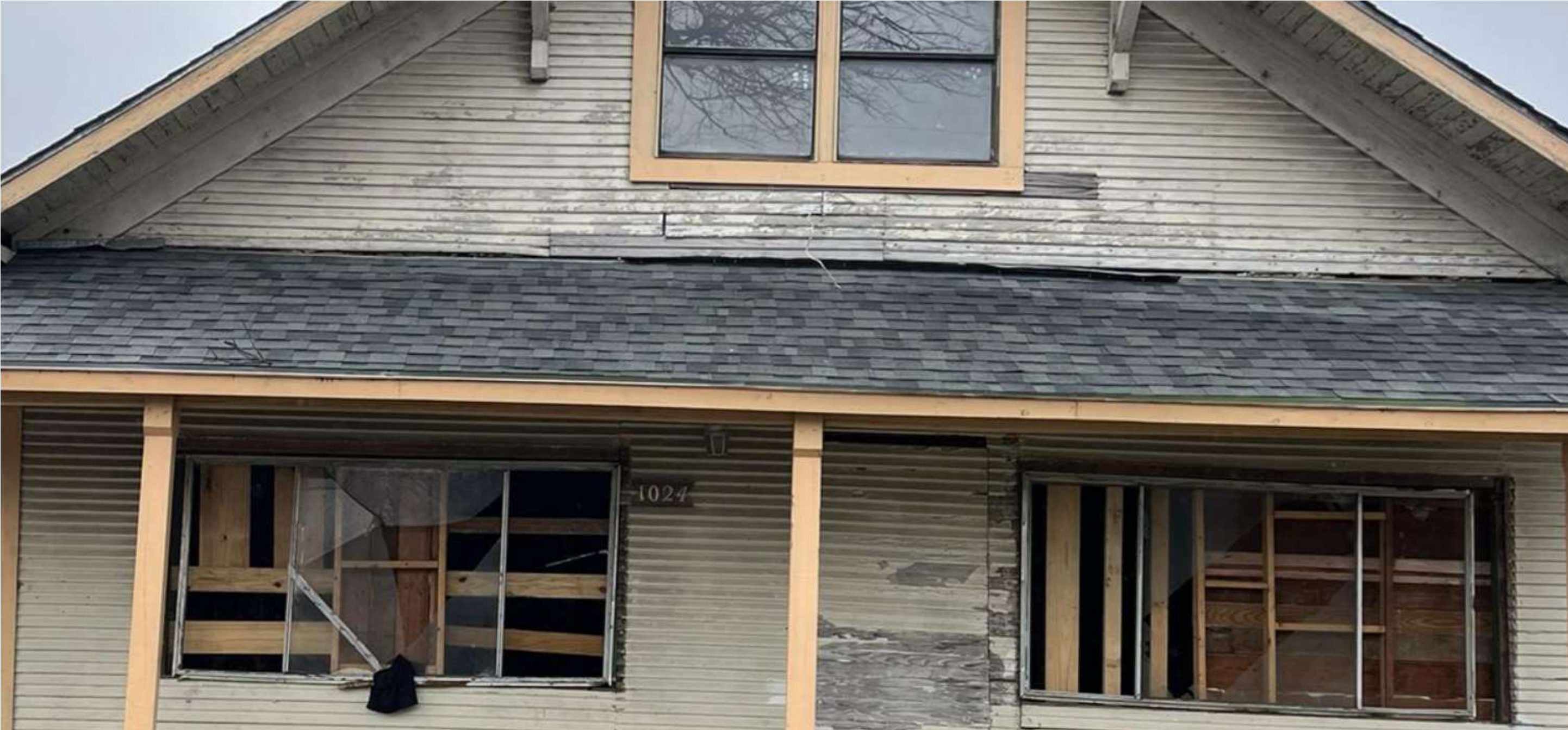
DAMAGED ALUMINUM WINDOWS
