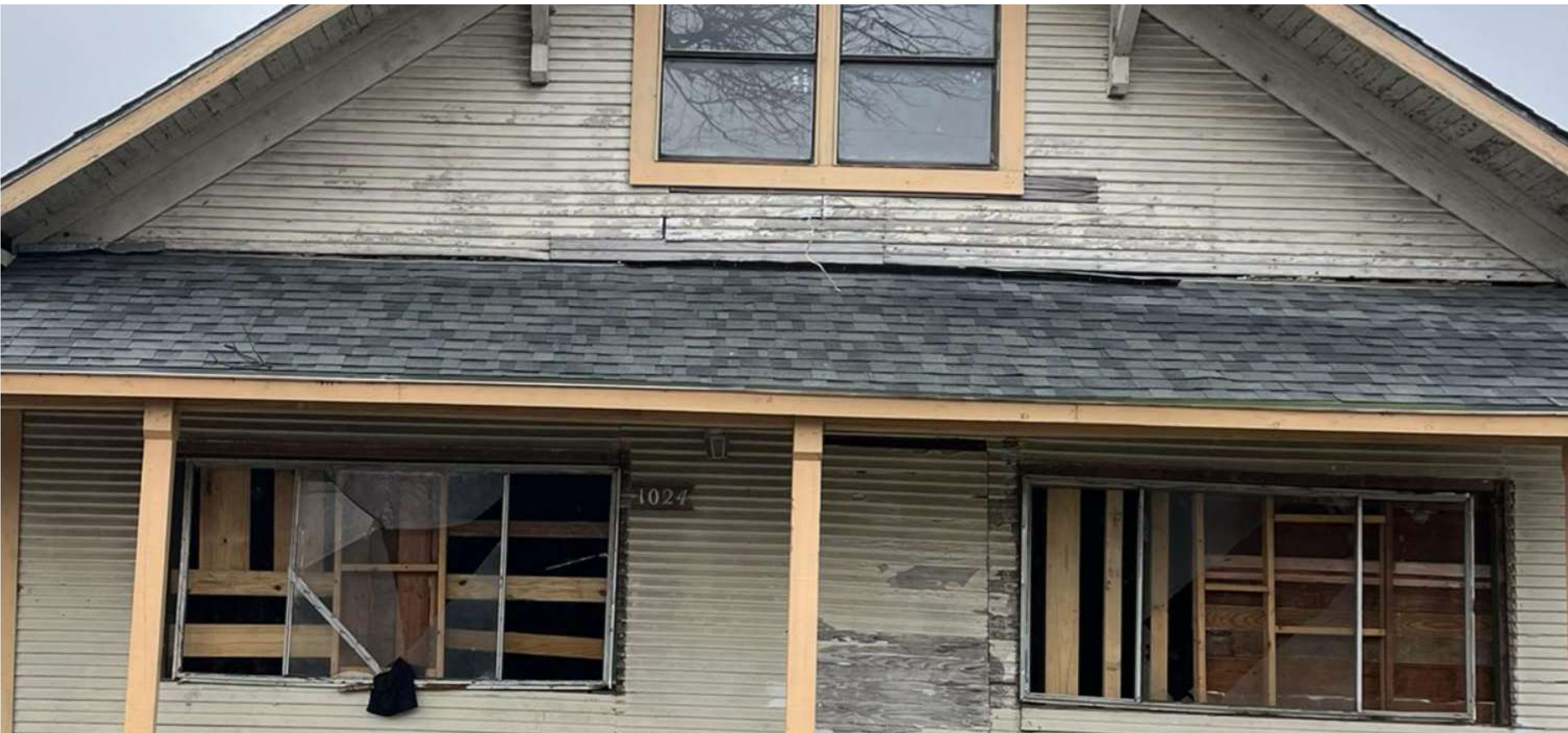
DAMAGED ALUMINUM WINDOWS
