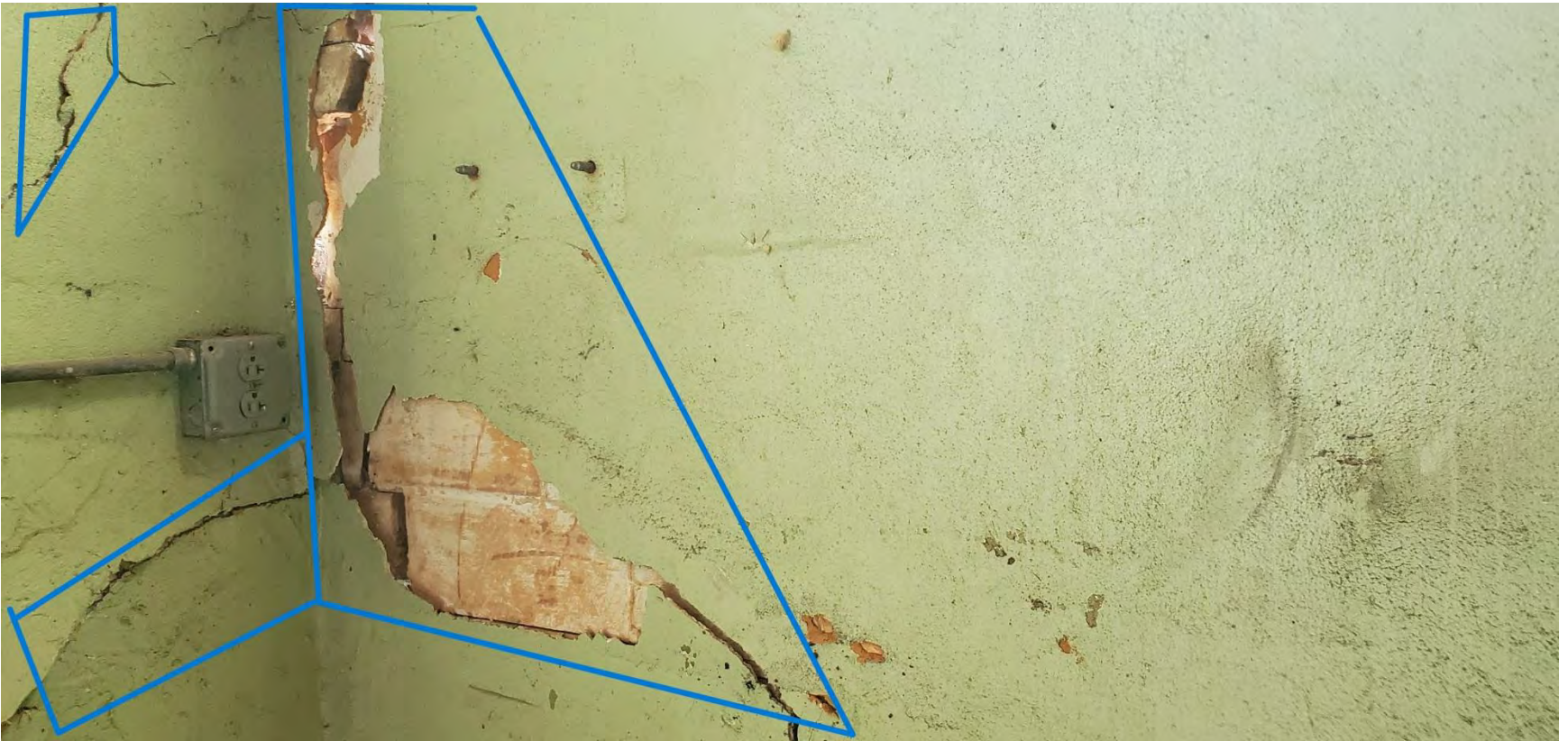
EXISTING WALL – VISIBLE GAPS – BUILDING MOVEMENT OVER TIME
