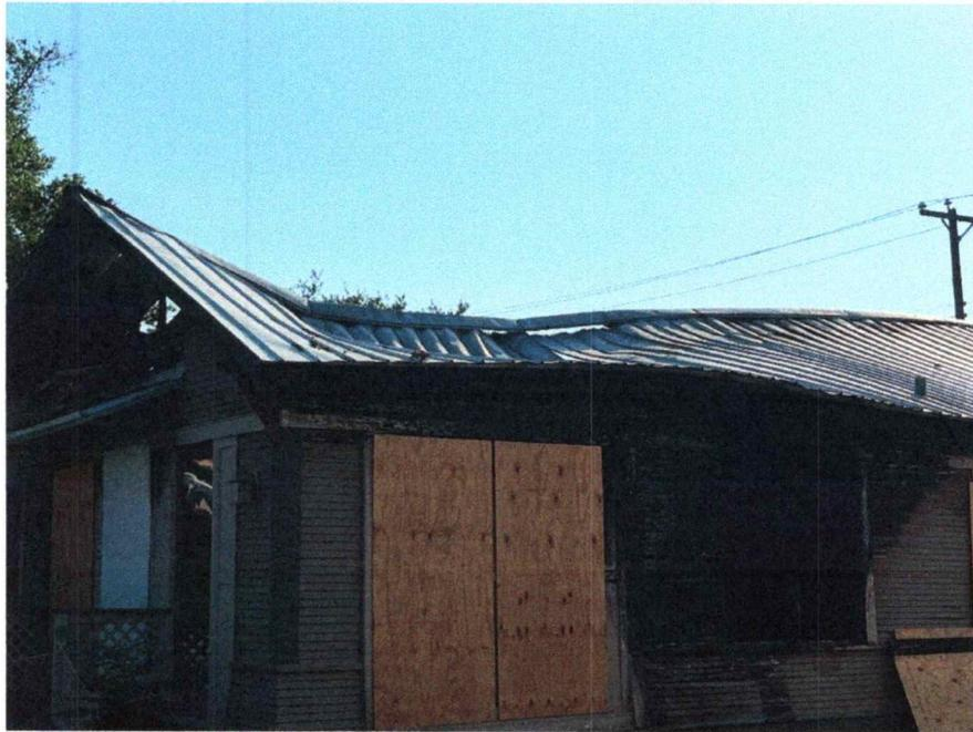
**Burned and Destroyed Roof Rafters with Much Roof Decking Gone**
