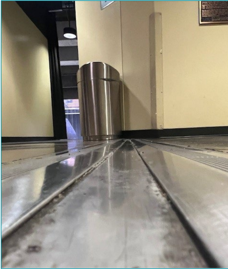
Existing Expansion Joints
