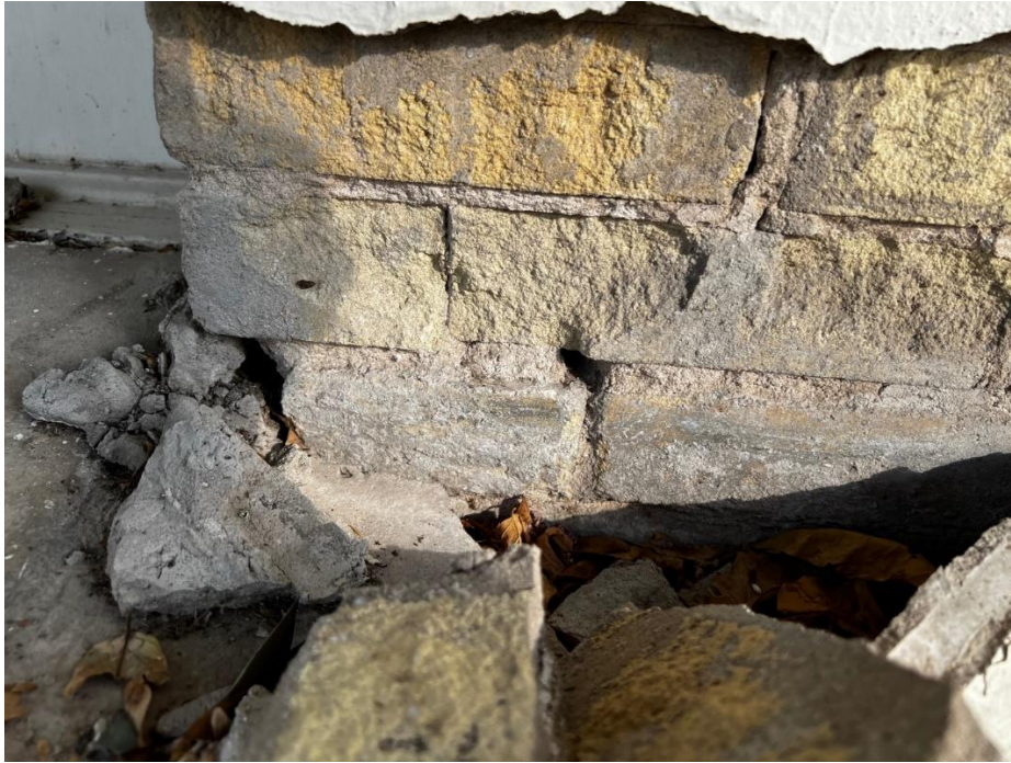
Plaster removal damages the original brick
