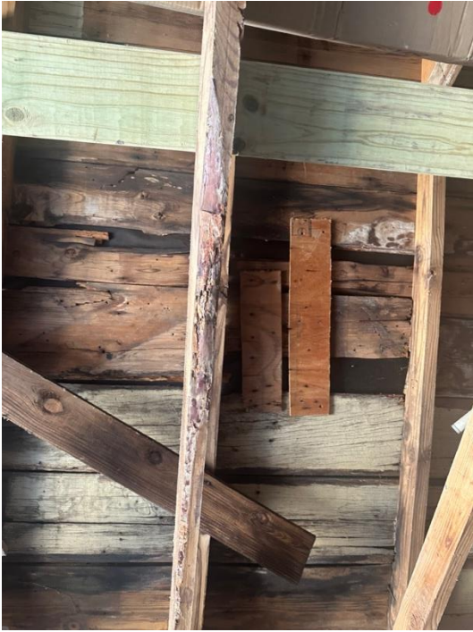
Interior of wood with rot and mold
