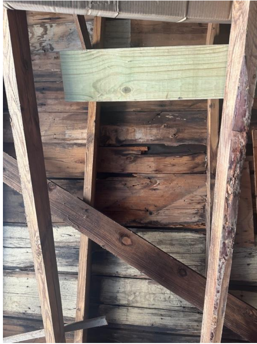
Interior of wood with rot and mold
