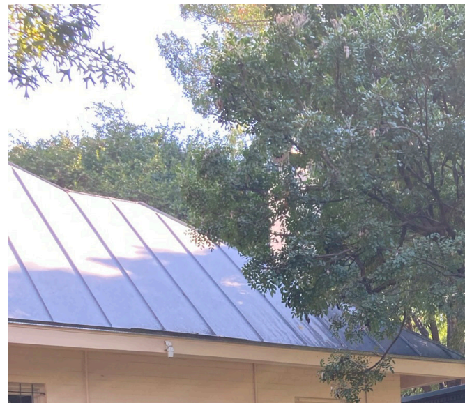
STANDING SEAM METAL ROOF
