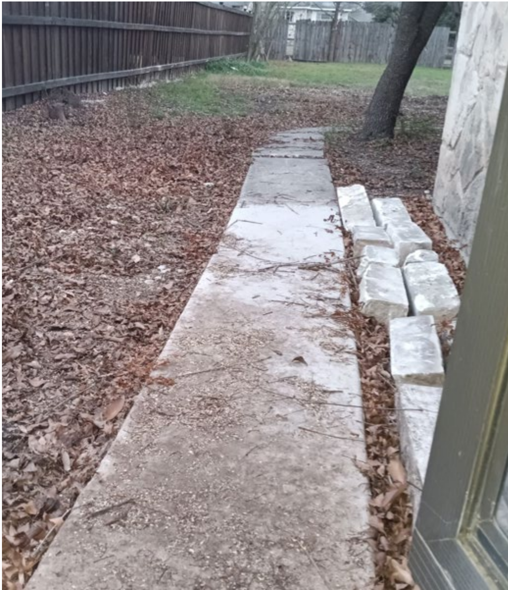
Sidewalks broken & slanted towards the house from the left side of the house
