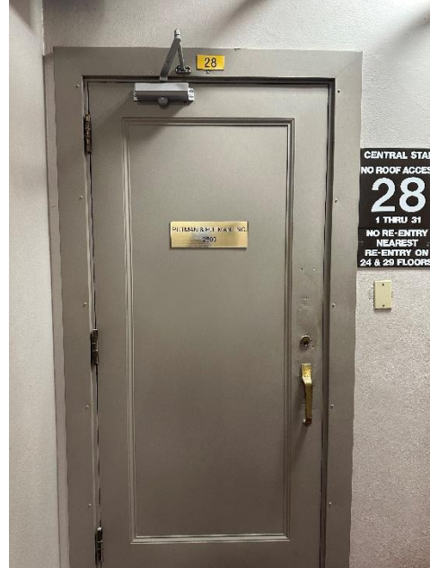
35. 28 th Floor – Example/ Original Fire-Rated Door at Existing Stair
