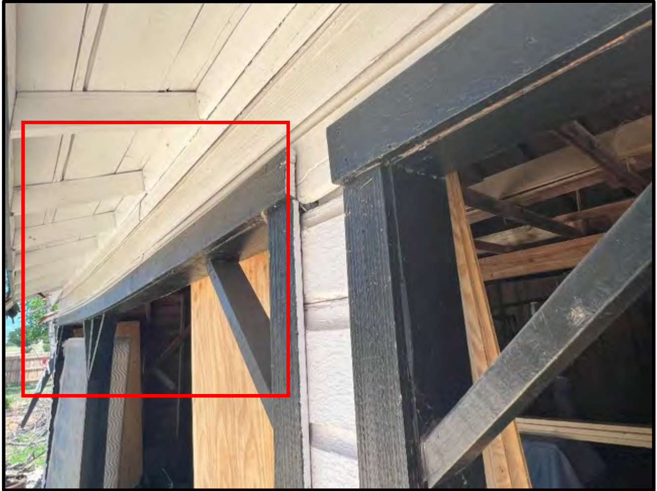
View of a deflection deformation of the opening header at the front (south) of the detached garage building. Note partially detached trim boards.
