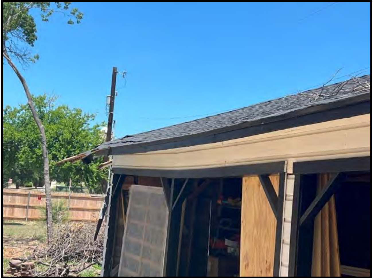
View of a deflection deformation of the opening header at the front (south) of the detached garage building.
