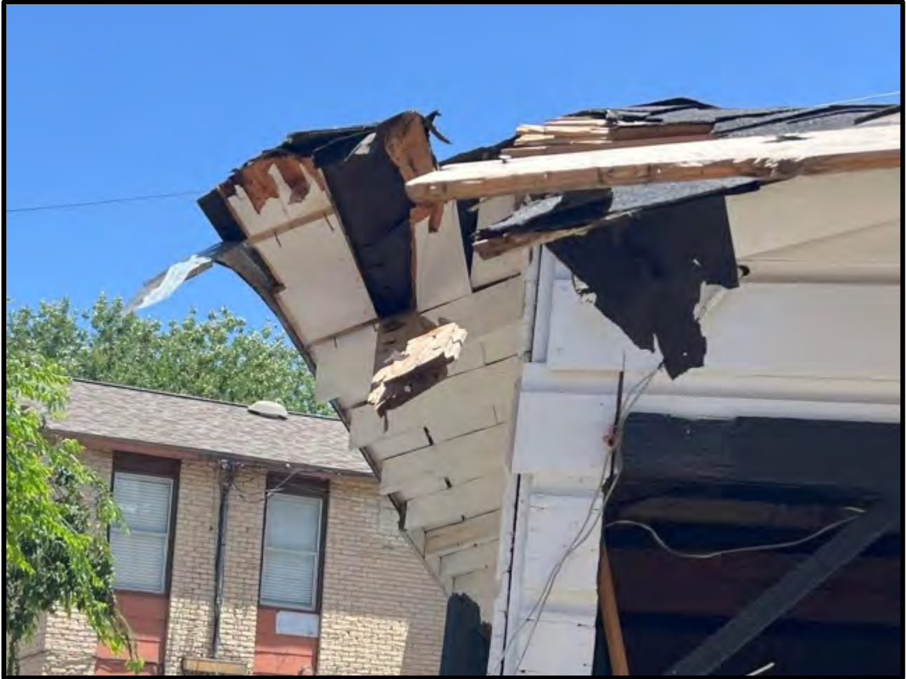
Close-up view of the impact area at the southwest corner of the detached garage building.
