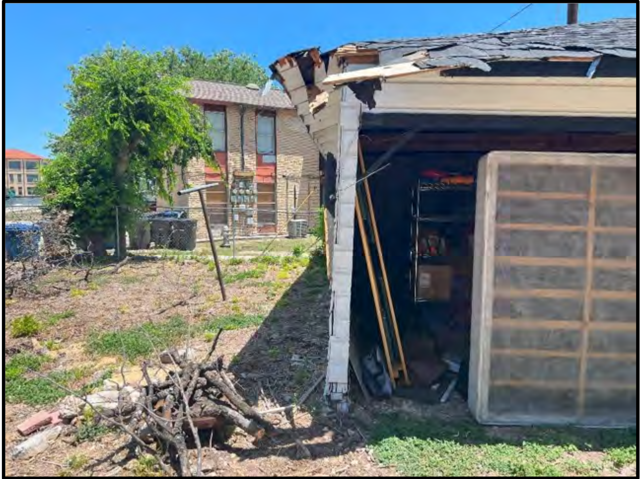
View of the impact area at the southwest corner of the detached garage building.
