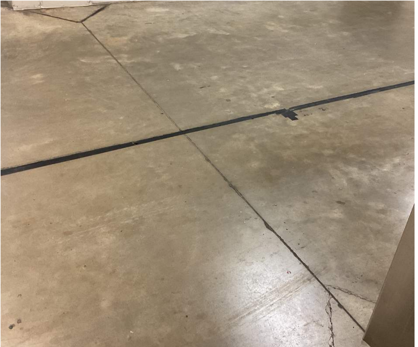
Existing Construction Joints at Field Level
